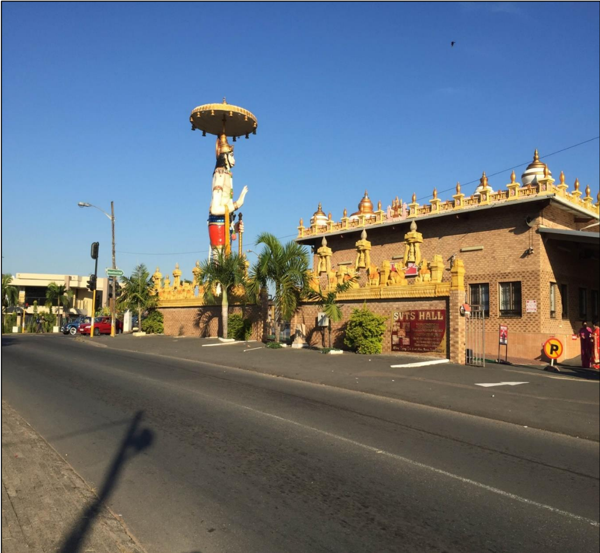
Plate 4: Conversion of residential to religious and community use (with or without planning consent) Source: Author
