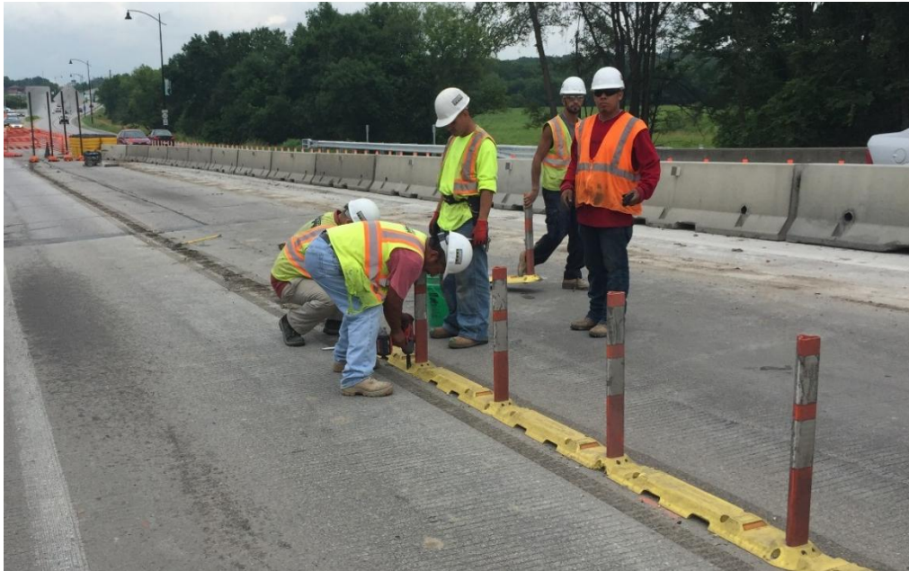
Figure 40. Temporary bollards being detached by workers
