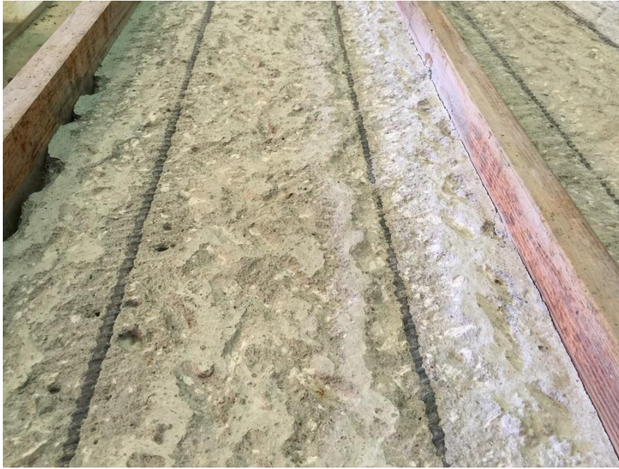
Figure 83. Positive bending flexural test specimen after roughening of substrate concrete (Case 1)
