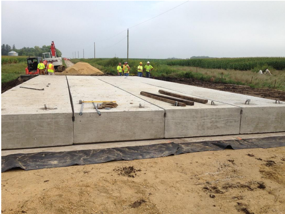
Figure 18. Four beams placed over the creek on the concrete abutments
