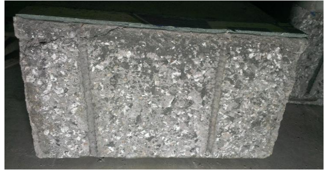
c) Bond interface (overlay concrete)
