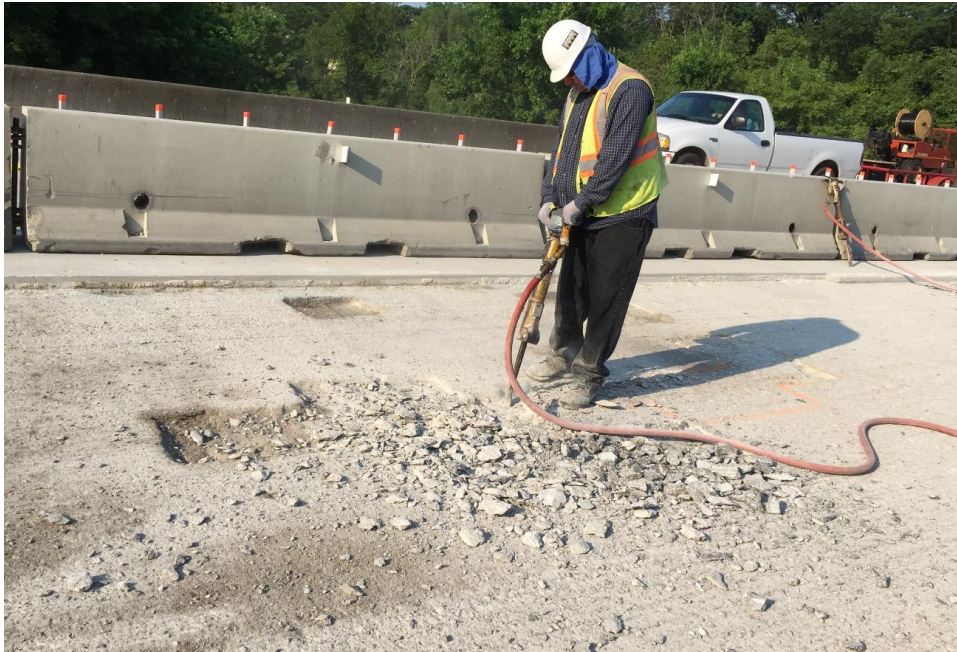
Figure 43. Removal of unsound concrete using jackhammer
