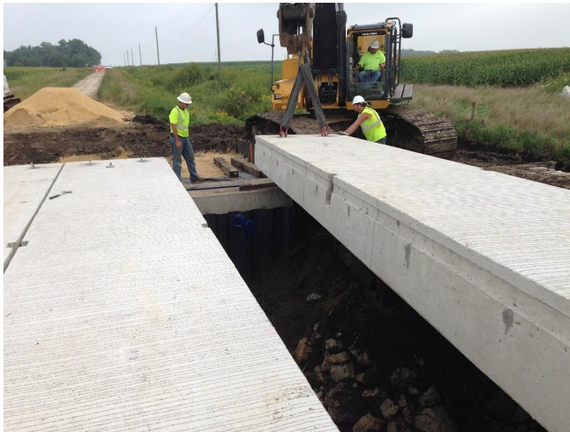
Figure 19. Fifth beam being moved to its position using backhoe
