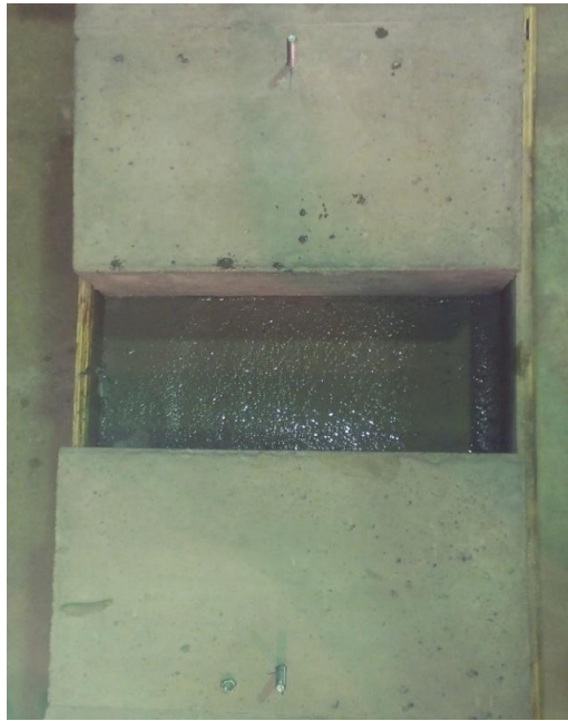
Figure 70. Push-out test specimen after overlay concrete placement
