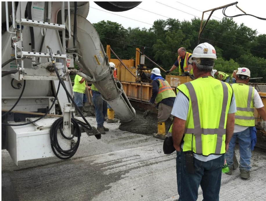
Figure 45. Ready-mixed concrete being placed on the deck
