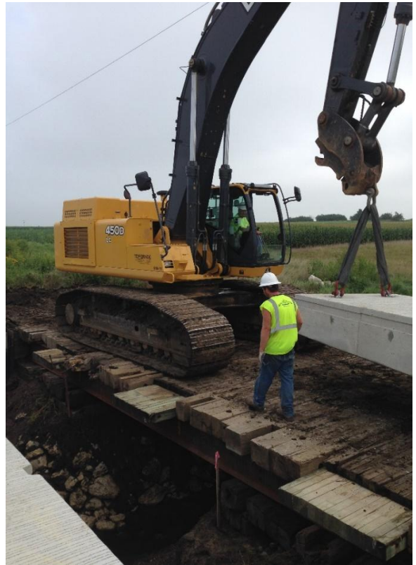
b) Beam move over the creek
