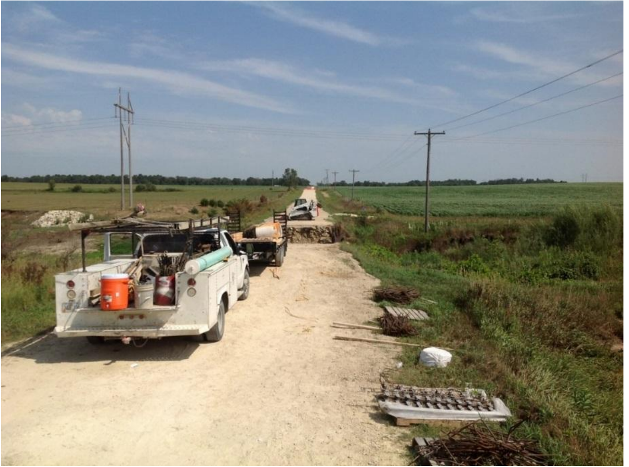
Figure 7. Construction job site
