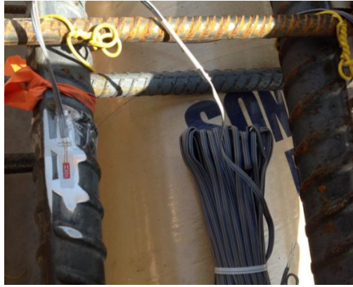
Figure 10. Gage installation on reinforcement
