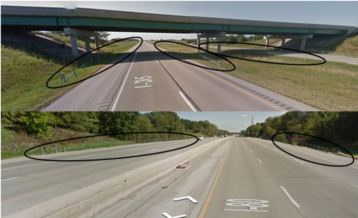
Figure 4: Cable barrier used to protect fixed objects (top); non-median cable barrier (bottom)
