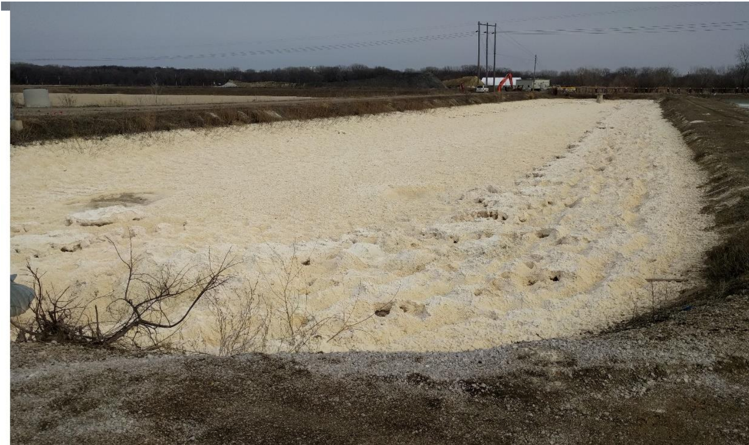
Figure 3. Lime sludge lagoon operated by Ames Water Treatment Plant
