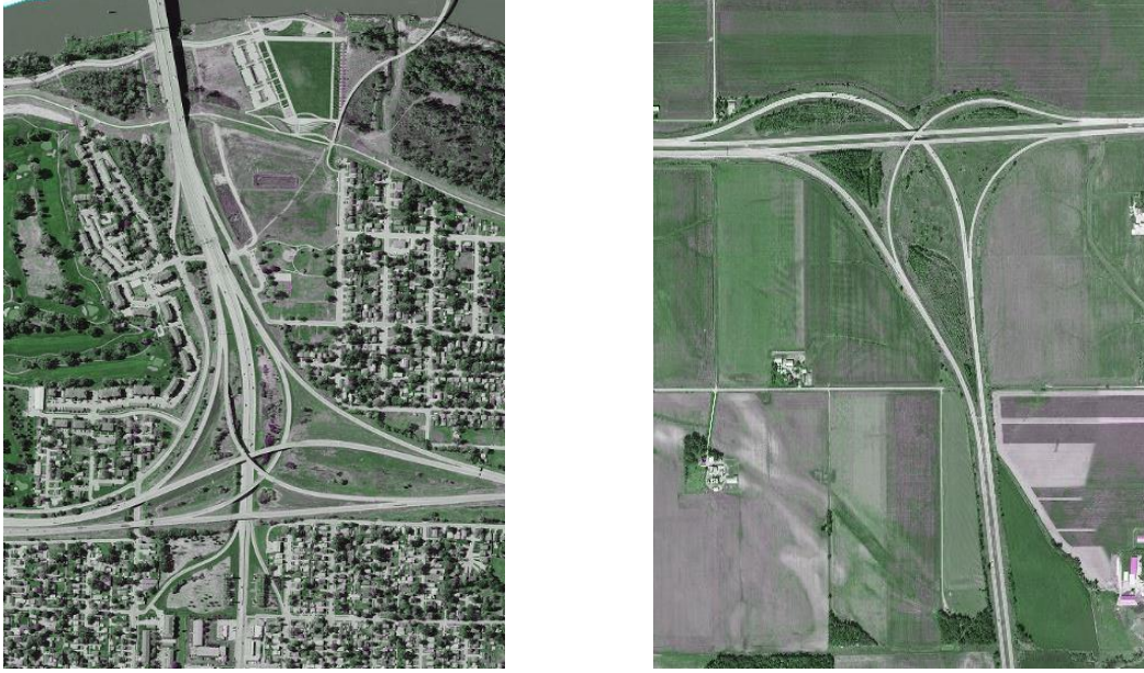
Figure 4: All Directional Interchange I-480/1-29 (left) and Three leg Directional Interchange I-380/US 20 (right)
