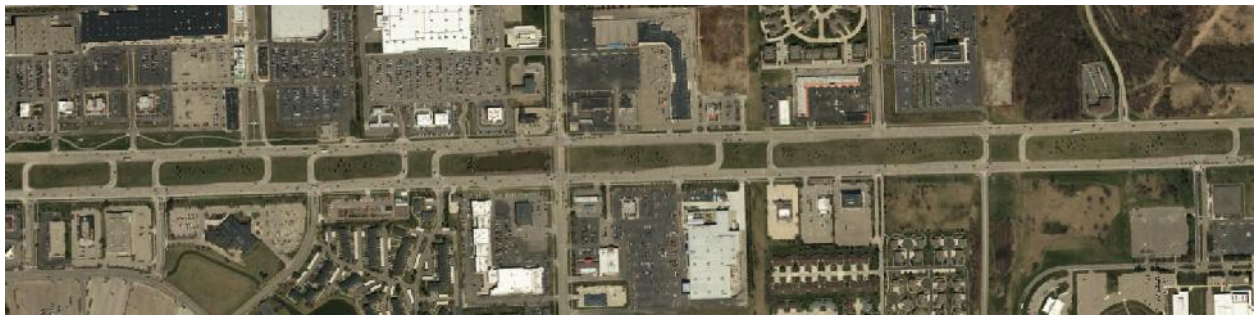
Figure 7. MUT Installations Along a Boulevard
