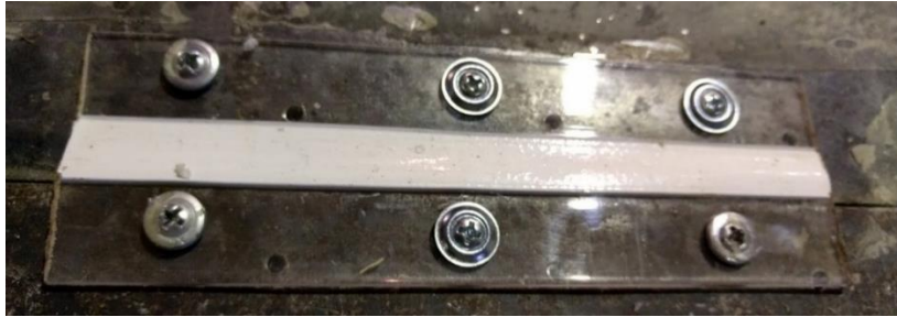
Figure 3.3 Shifted rubber bolted to the formwork to achieve 90° angle
