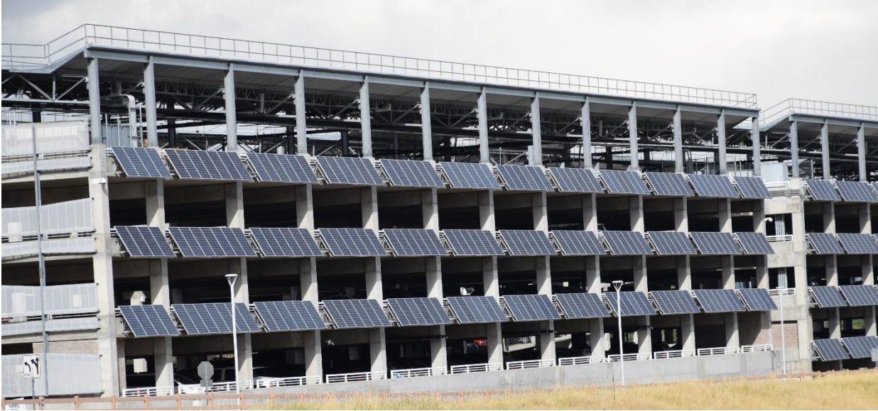
Figure 1.1 PV modules mounted to the wall of a multistory parking at NREL, CO
