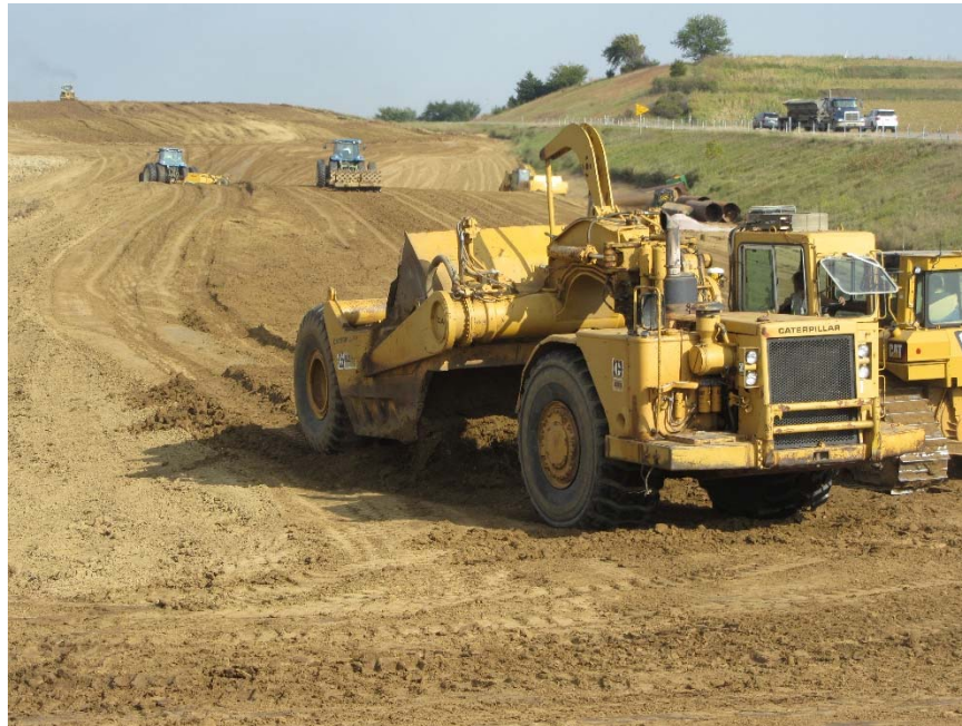
Figure 141. Woodbury County Project 9: Caterpillar 631D motor scraper used to collect and place loose fill materials
