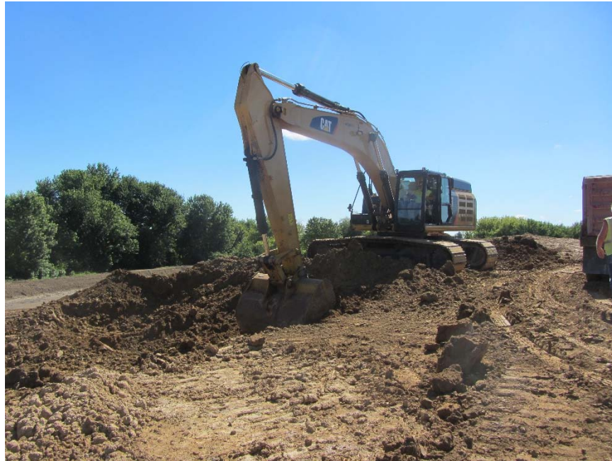
Figure 126. Scott County Project 8: Caterpillar 349E used to excavate materials from borrow source
