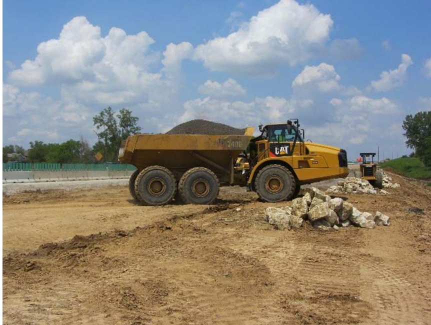
Figure 22. Polk County Project 1: Caterpillar 740B dump truck used to place loose fill materials
