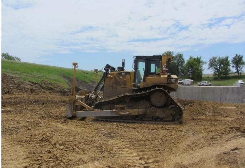
Figure 38. Warren County Project 2: Caterpillar D6T dozer used to control lift thickness
