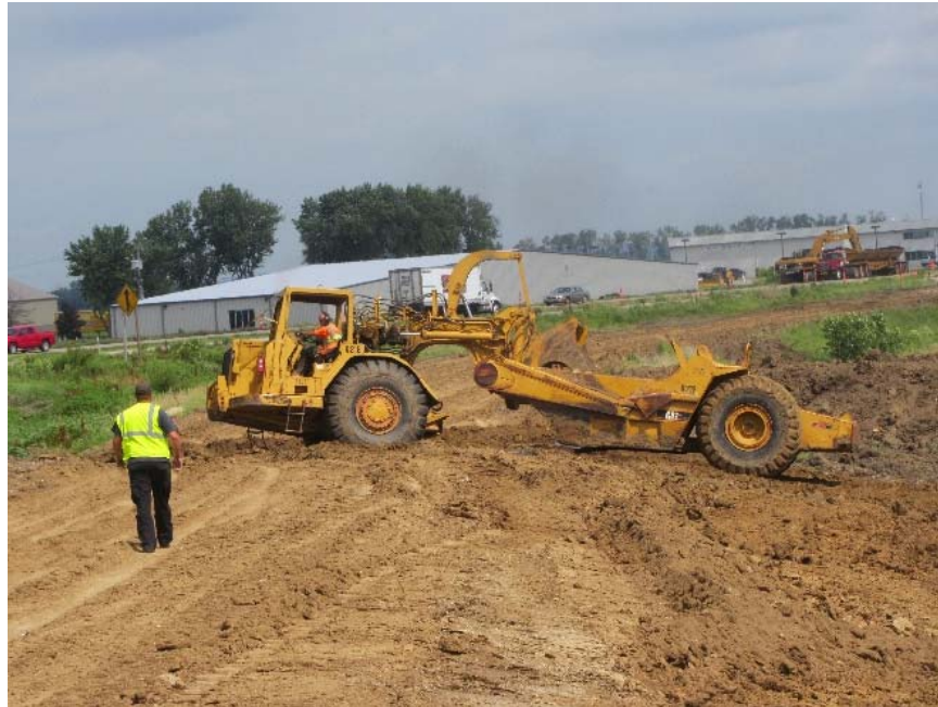
Figure 88. Mills County Project 5: Caterpillar 621E scraper used to collect and place loose fill materials
