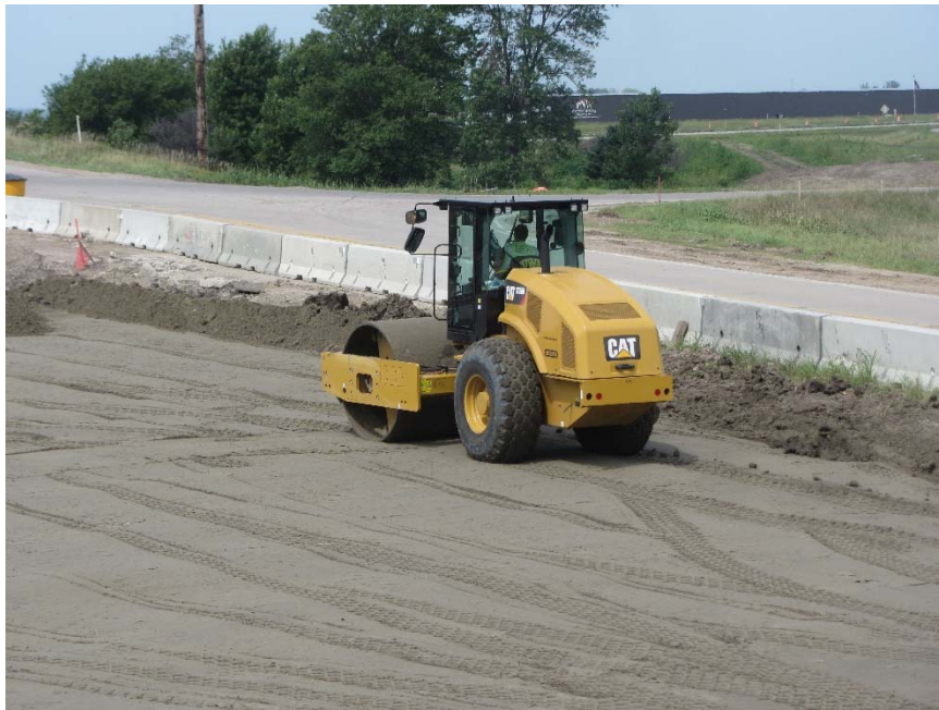
Figure 114. Woodbury County Project 7: Caterpillar CS56B vibratory smooth drum roller used for soil compaction
