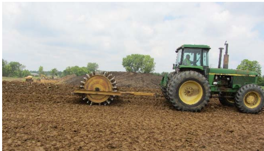
Figure 75. Linn County Project 4: Sheepsfoot roller used for soil compaction
