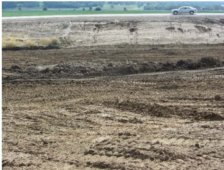
Figure 91. Mills County Project 5: Very wet materials in the center of the construction site
