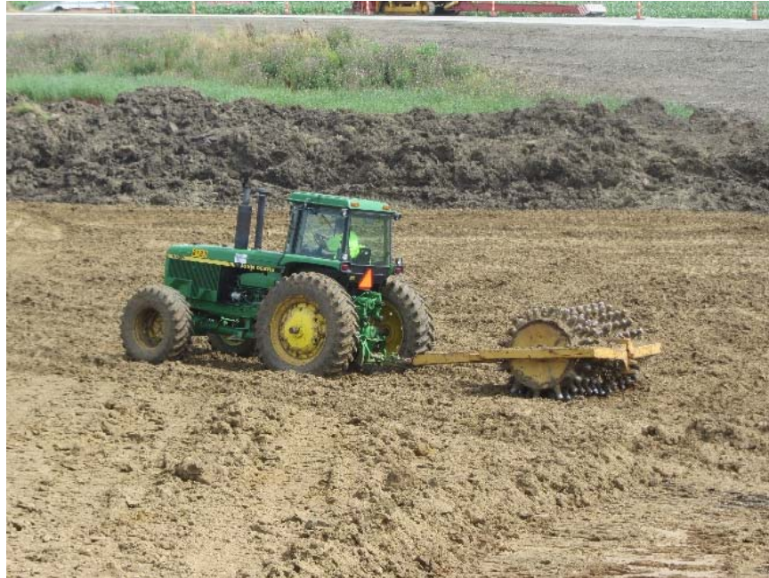
Figure 90. Mills County Project 5: Sheepfoot roller used for soil compaction
