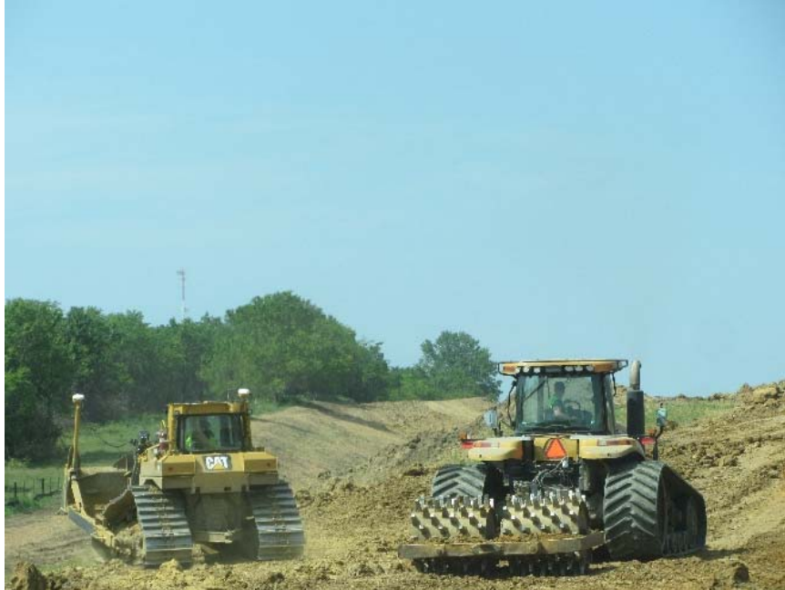
Figure 40. Warren County Project 2: Sheepfoot roller used for soil compaction
