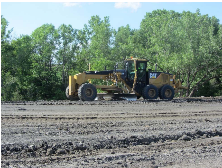
Figure 56. Linn County Project 3: Caterpillar 14M motor grader used to level the embankment surface
