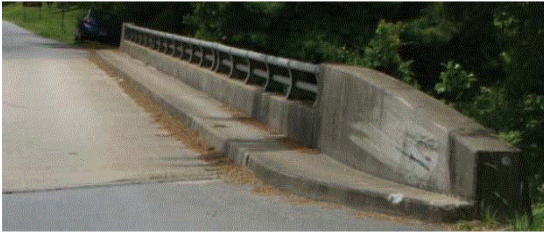
Figure 11: Unshielded Bridge Rail End
