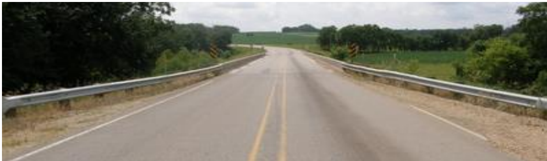
Figure 1: County Highway Bridge over the South Fork of the Iowa River in Hardin County, Iowa
