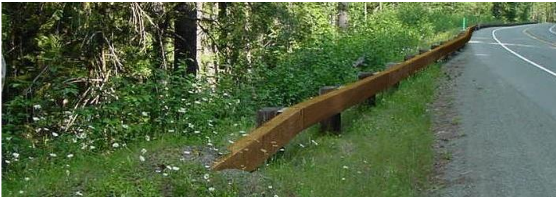
Figure 10: Example of a traditional SBT guardrail with buried in backslope end-treatment
