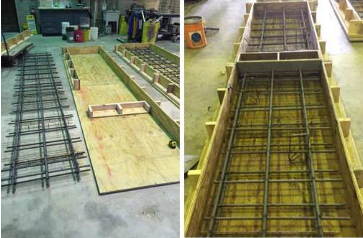
Figure 3-11. Steel Reinforcement and Formwork Fabrication
