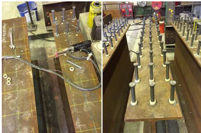
Figure 3-28. Placement of Shear Studs
