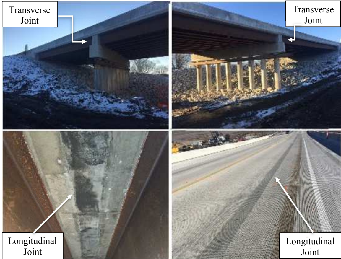
Figure 3-3. Constructed Little Silver Creek Bridge
