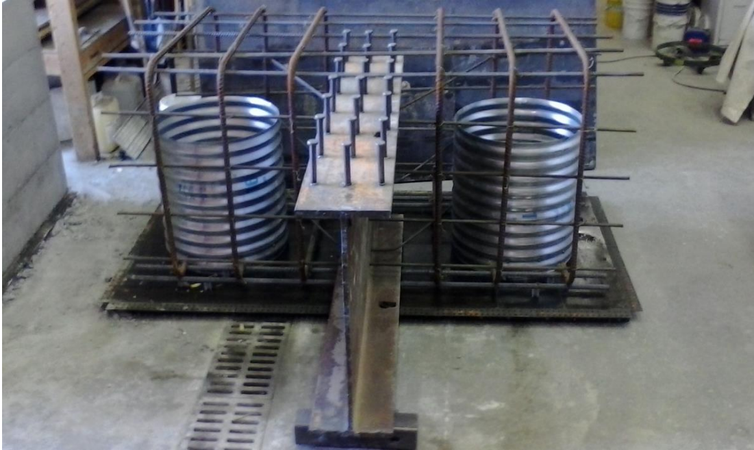
Figure 43. Integral diaphragm rebar cage
