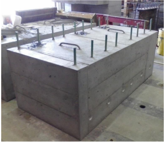
Figure 24. Grouted coupler pile cap
