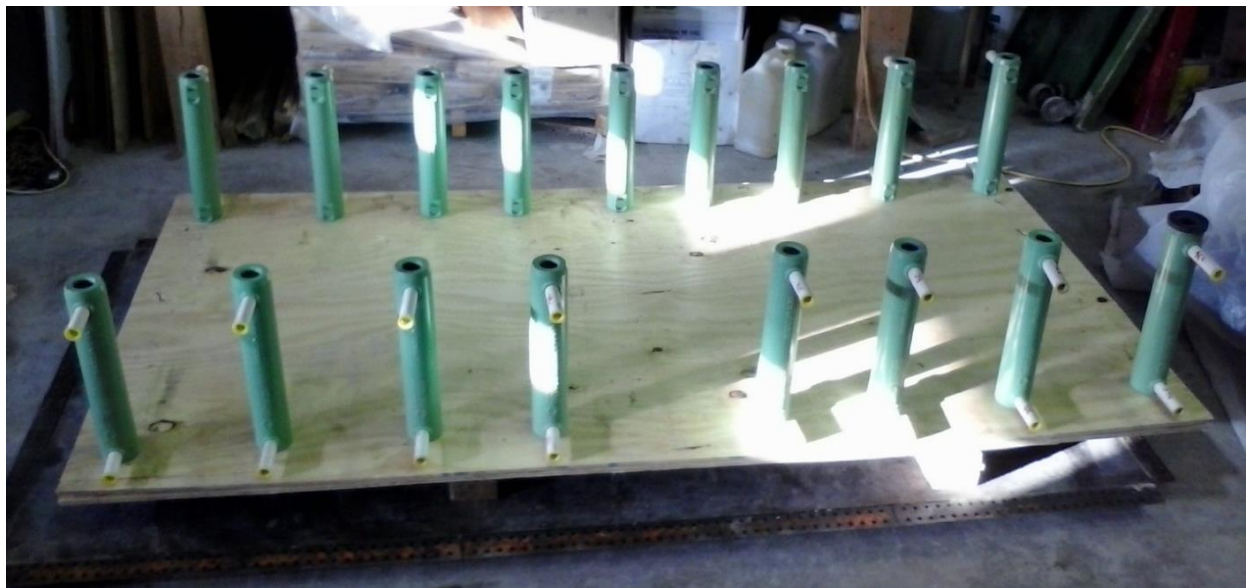
Figure 25. Grouted coupler template
