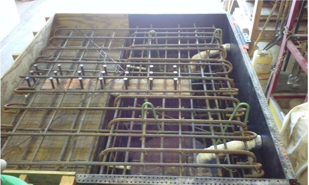
Figure 45. Integral diaphragm deck rebar
