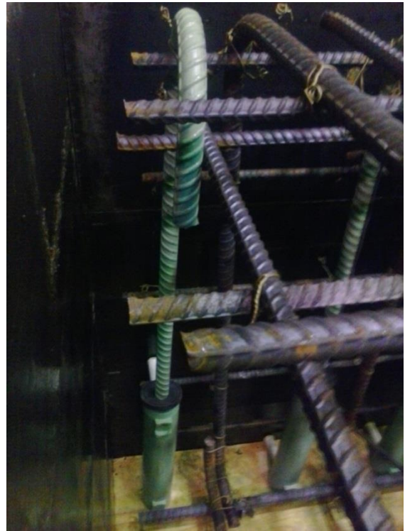
Figure 27. Grouted coupler and rebar
