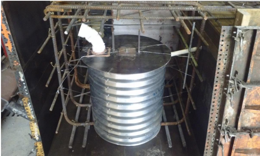
Figure 44. Side view of CMP void
