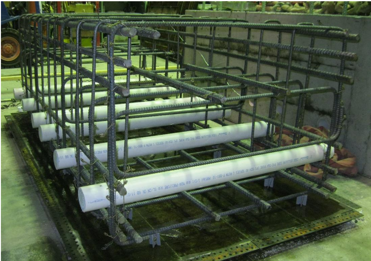
Figure 37. Pile cap rebar cage
