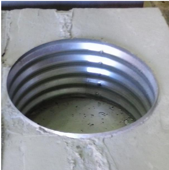
Figure 39. CMP void in pile cap
