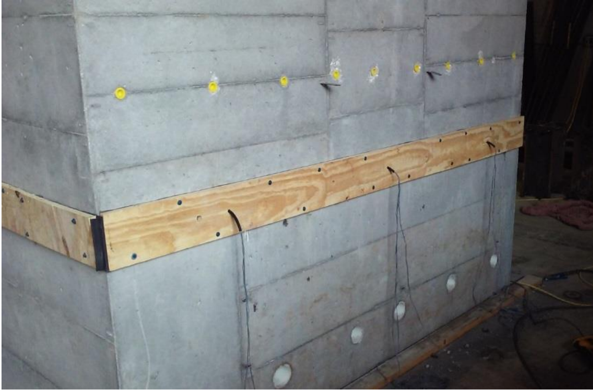
Figure 33. Grout bed formwork
