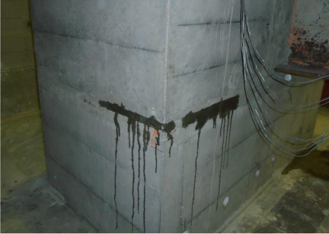
Figure 53. Bleed water passing through the grout bed
