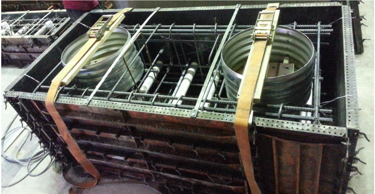
Figure 38. Pile cap rebar, formwork and CMP
