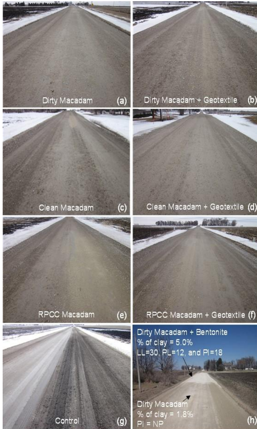
Figure 4.7. Surface conditions of (a through g) the MSB and control sections during the first thawing period (photos taken March 11, 2014), and (h) dirty macadam sections with and without the bentonite surface treatment during the second thawing period (photo taken March 28, 2015).
