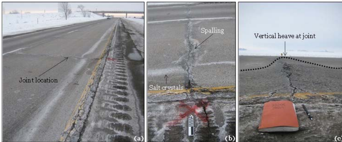
Figure 4.1. Field pictures showing (a) the EB on US 30, (b) joint deterioration with spalling, and (c) vertical heave at joint location.
