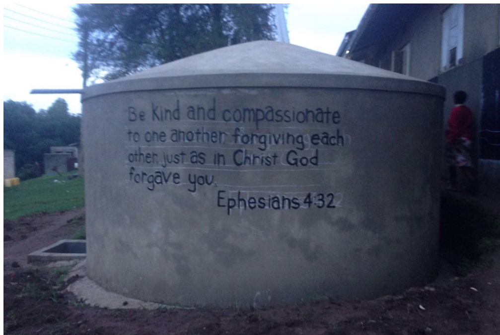
Figure 4: 30,000 Liter Brick by Brick Rainwater Harvesting Tank constructed for Bikungu Primary Teacher's College.
