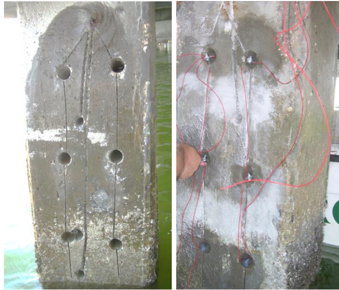
Figure 10.13 Instrumented face for hybrid FRP-CP Pressure bagged repair (2008)
