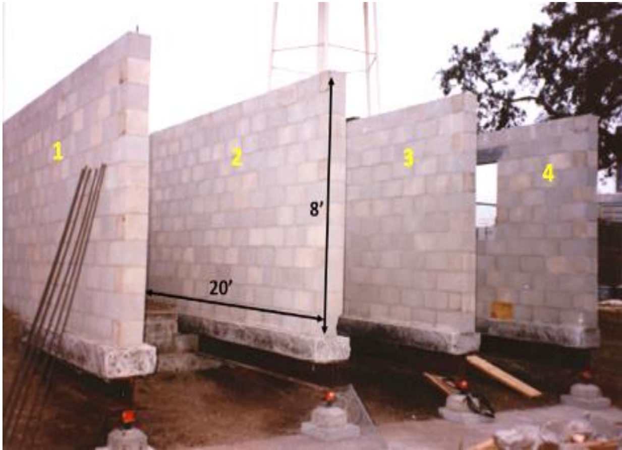
Figure 9.2 Walls labeled 2 and 3 were repaired using CFRP and tested
