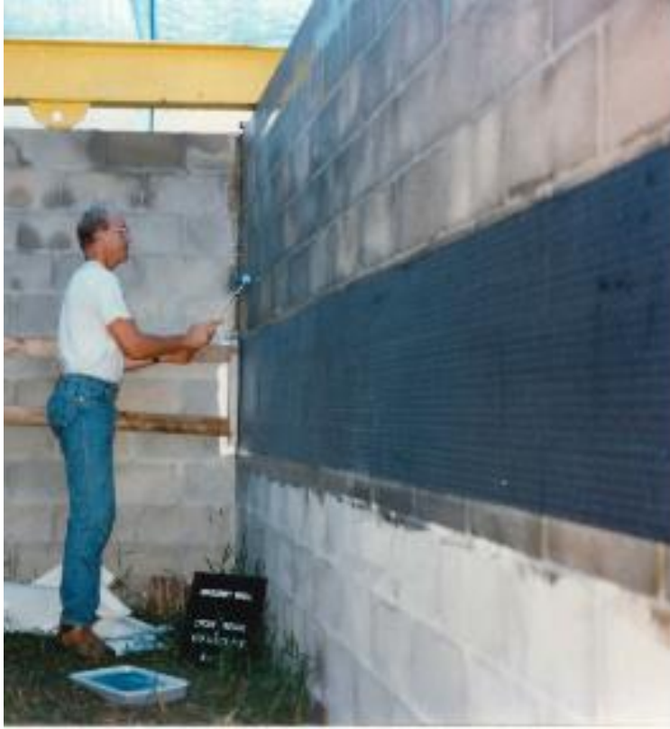
Figure 9.5 CFRP installation on epoxy wetted surface
