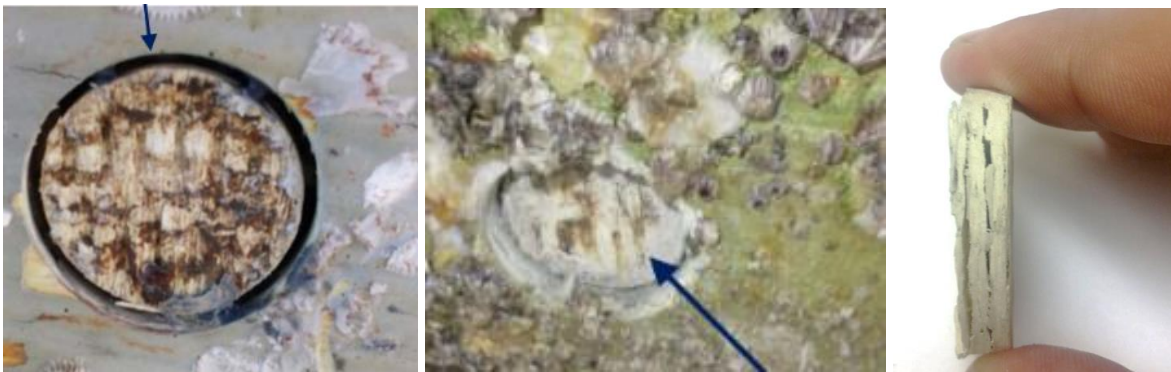
(b) Marine growth between FRP layers and voids between FRP layers
