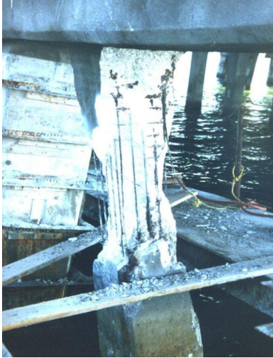
Figure 2.2 Pre-repair removal of chloride contaminated concrete.
