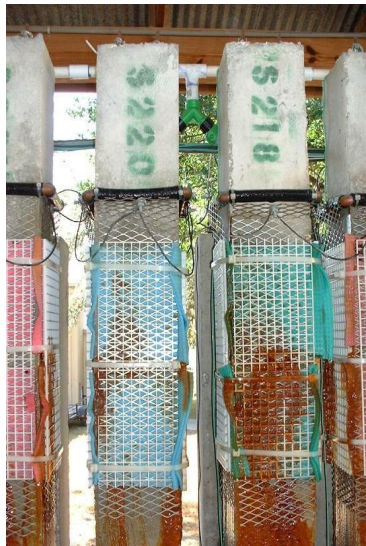
Figure 2.3 Corrosion cells instrumented on piles.
