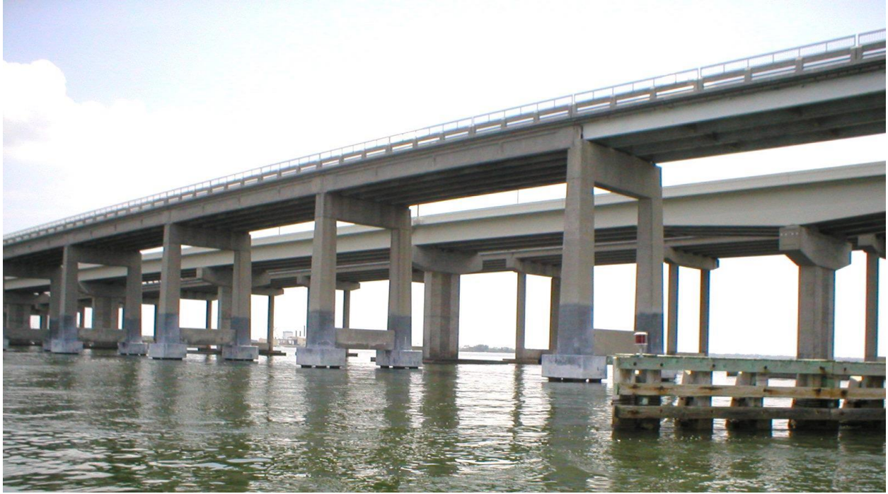
Figure 1.2 Cap and column configuration - Gandy Bridge adjacent to the navigation channel.
