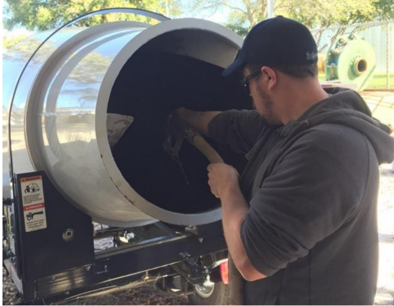
Figure 3.14. Concrete mixing for phase 2 shafts.
