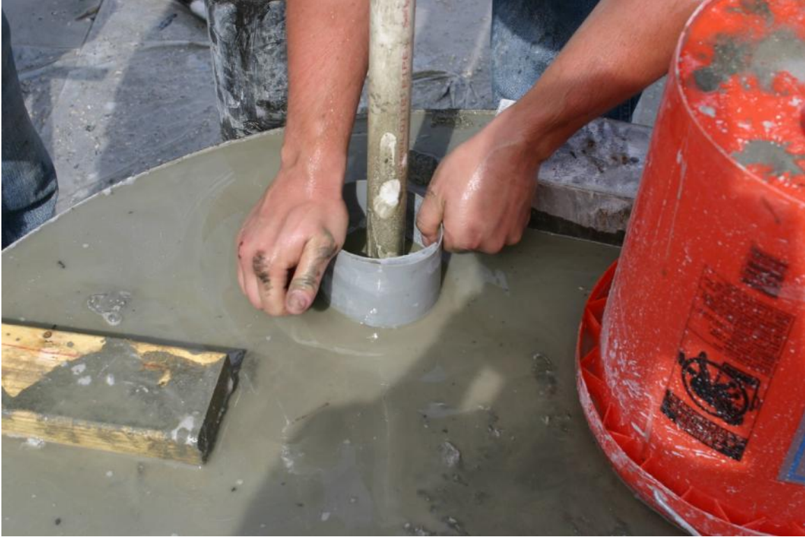
Figure 4.16. Debonding plastic sleeves on top 8in of the sockets.
