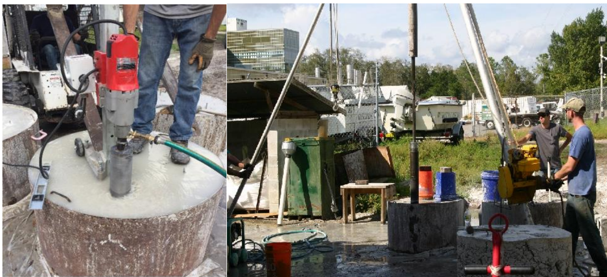
Figure 4.9. Pre-drilling (left) and driving the casing (right).
