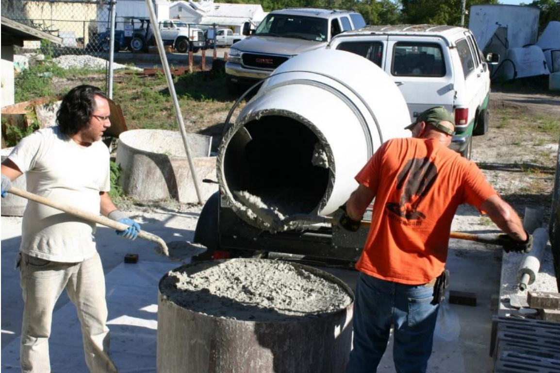
Figure 4.2. Casting of simulated limestone bed.
