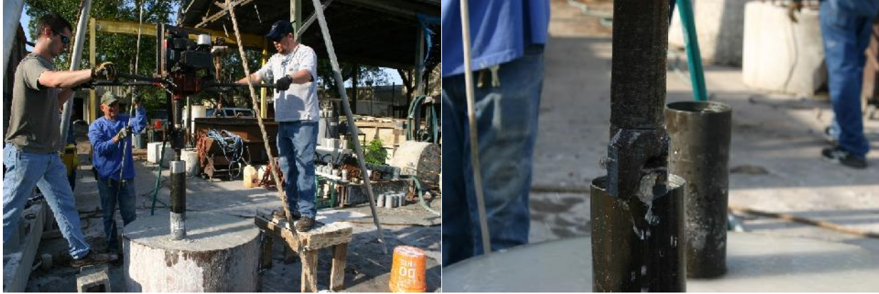
Figure 4.11. Rotatory casing installation (left) and drill bit (right).
