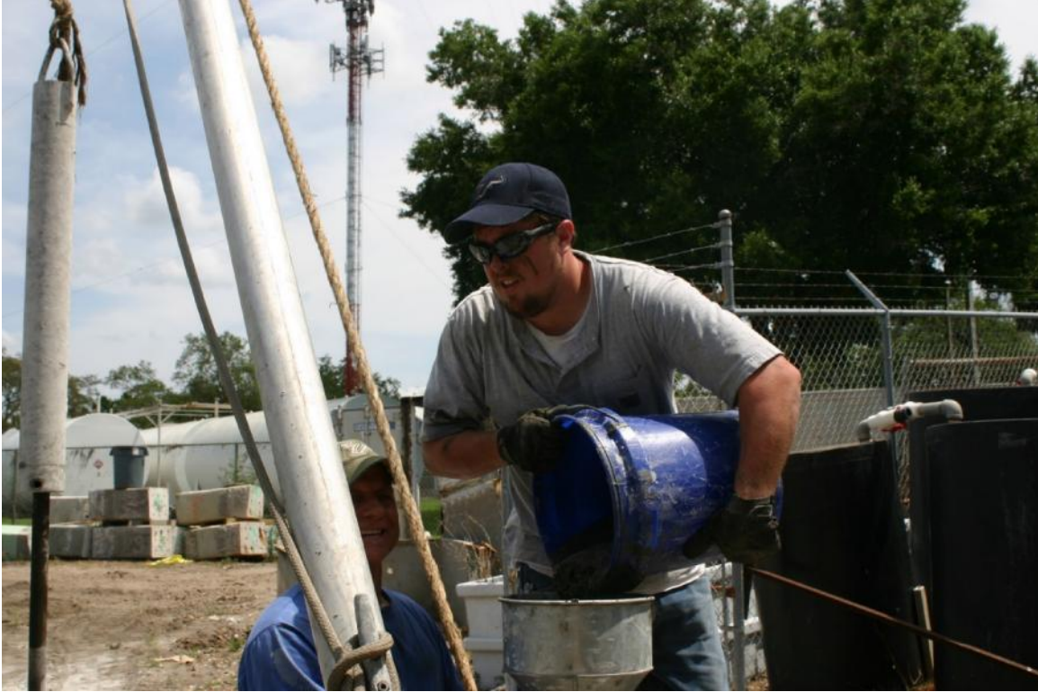
Figure 4.14. Concrete casting on the rock sockets.
