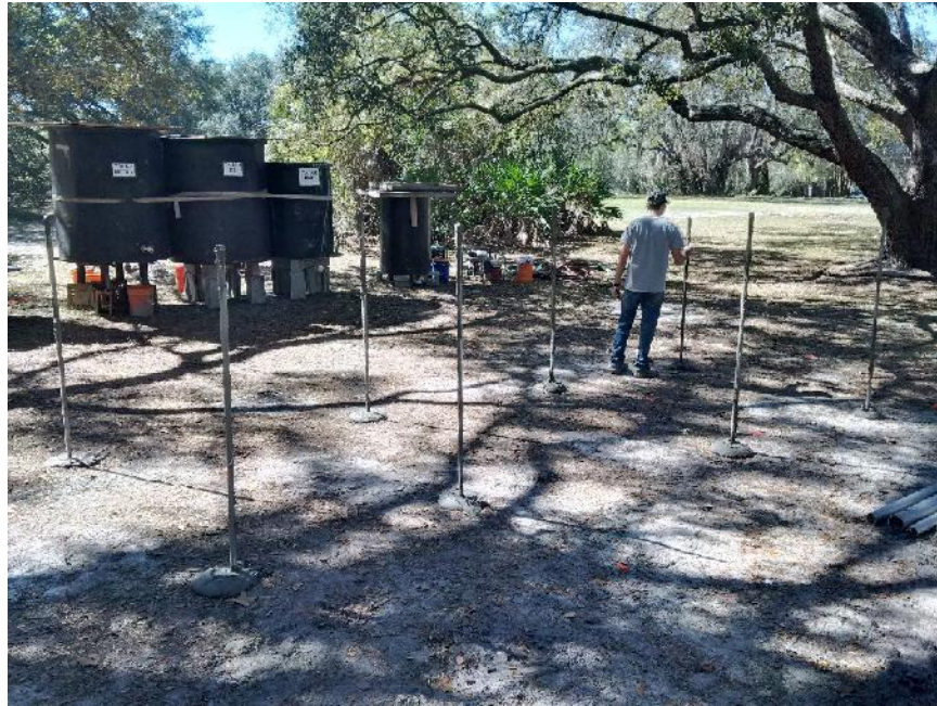
Figure 5.1. Partial view of freshly concreted test shafts.
