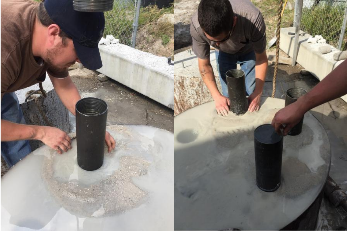
Figure 4.12. Cuttings replacement on the outer perimeter of the casings.
