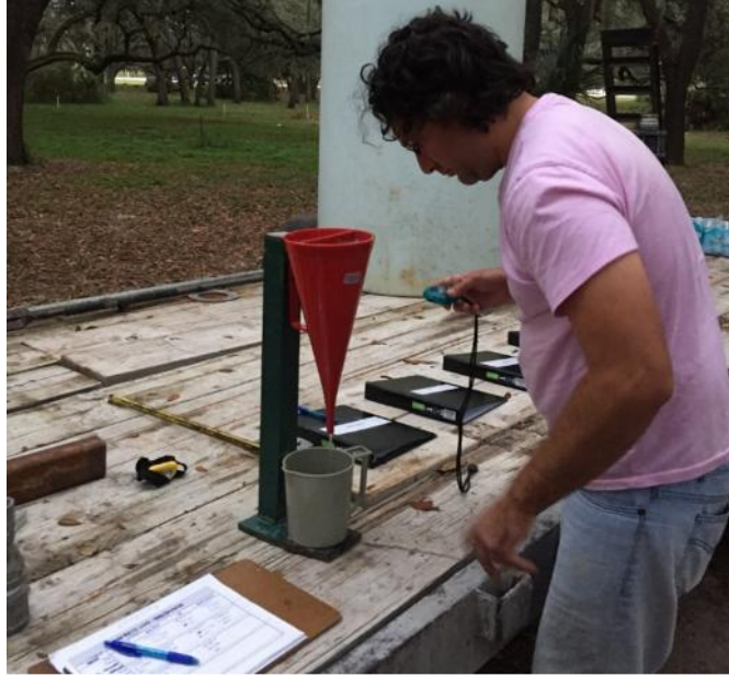
Figure 3.11. Viscosity measurement during the construction of phase 2 shafts.
