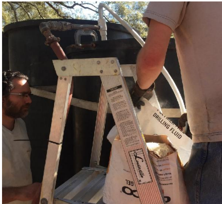
Figure 3.5. Bentonite slurry mixing.
