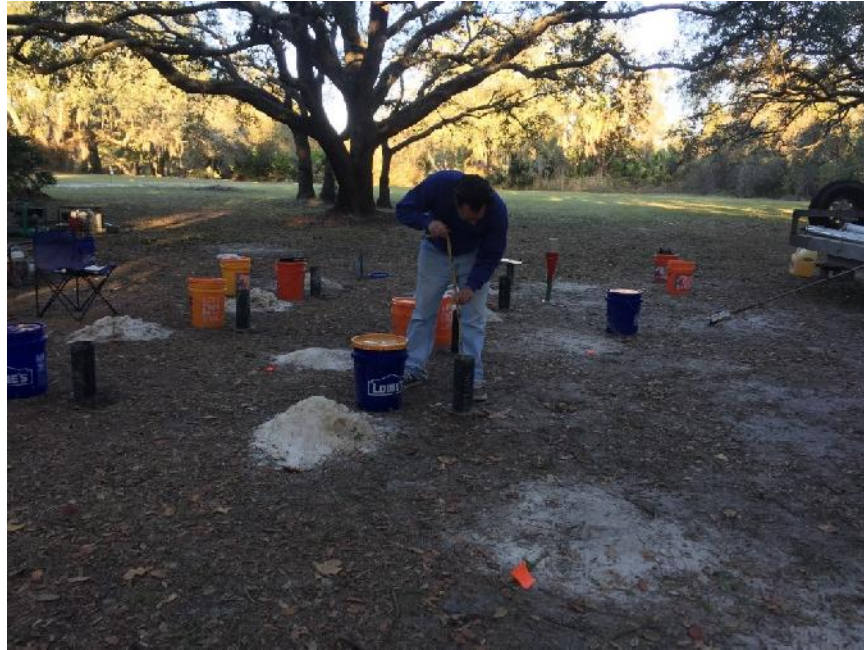
Figure 3.23. Monitoring of fluid level on phase 2 shafts.
