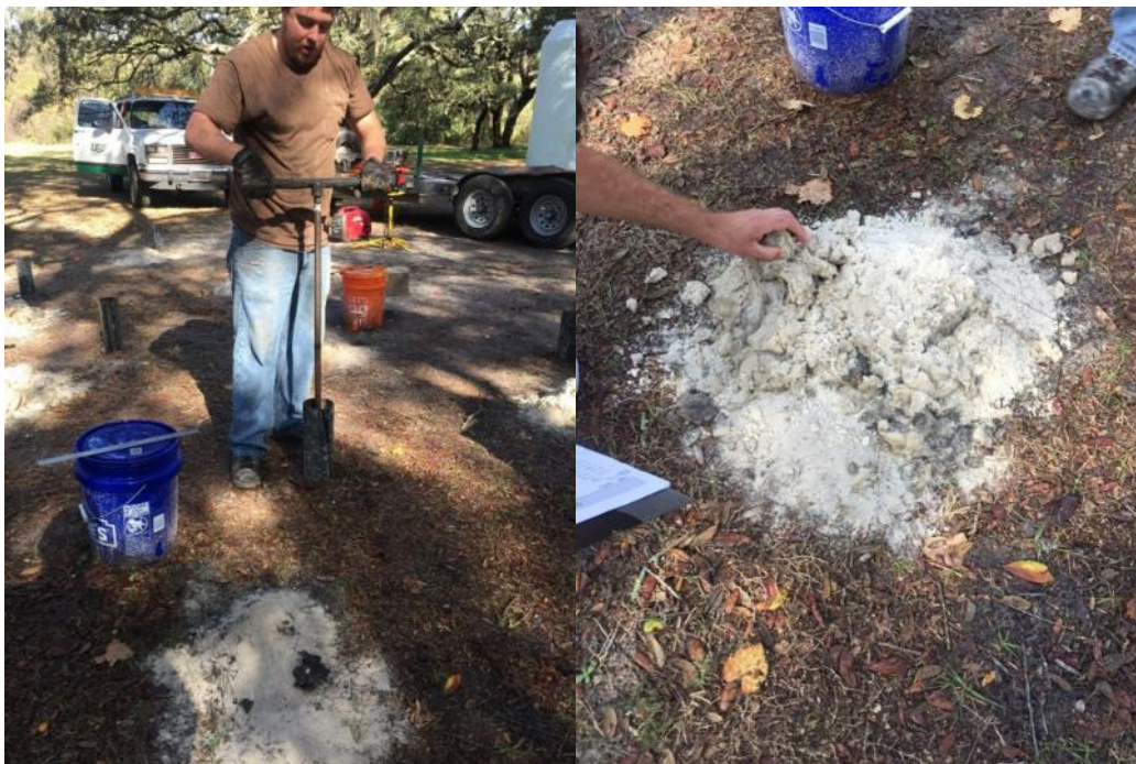
Figure 3.12. Phase 2 shafts excavation (left) and predominant silty-sand soil (right).
