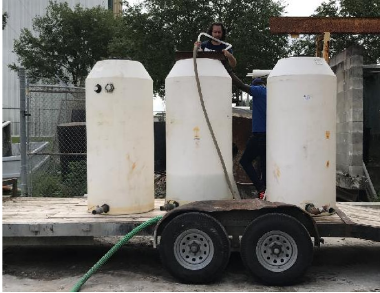
Figure 3.9. Phase 3 shafts slurry mixing.
