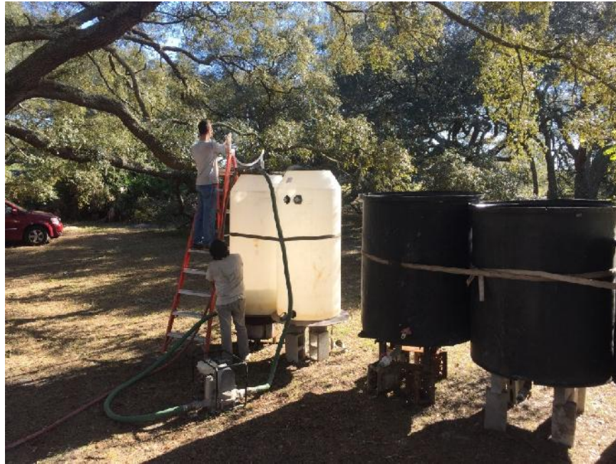
Figure 3.6. Cetco polymer mixing.
