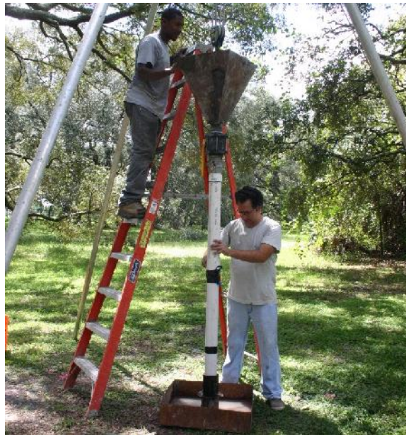
Figure 3.13. Illustration of concrete placement.
