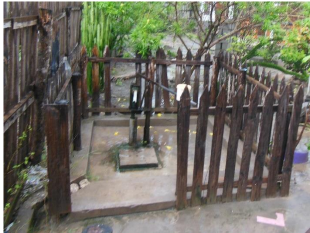
Figure 2.6 Examples of a full well apron around a Malagasy Pitcher Pump. (Picture taken by the author.)
