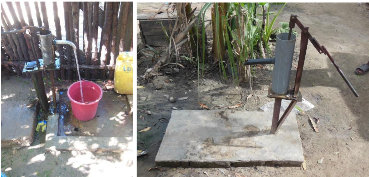
Figure 2.5 Examples of half well aprons around Malagasy Pitcher Pumps. (Pictures taken by the author.)
