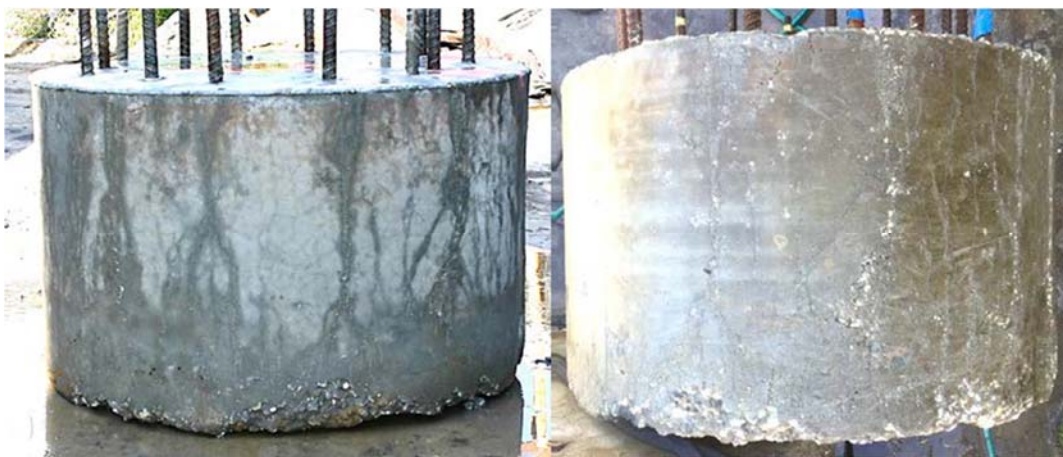
Figure 2.12 Shaft 6: f'c 4358 psi; drilled shaft mix, water cast, smooth with minor channeling
