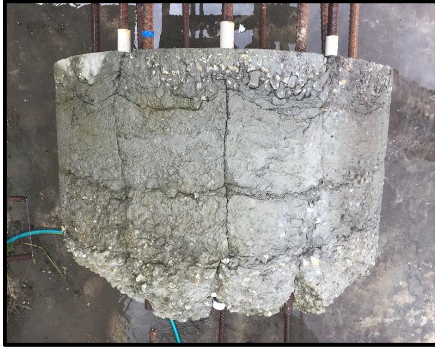
Figure 5.1 Reflective quilting exhibited in a drilled shaft test specimen
