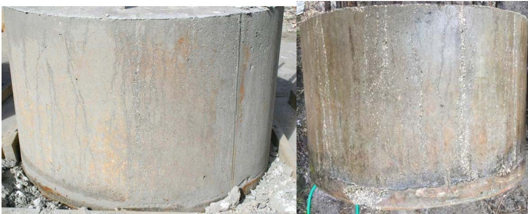
Figure 2.29 Shaft 23: self consolidating concrete, water cast, smooth minor channeling
