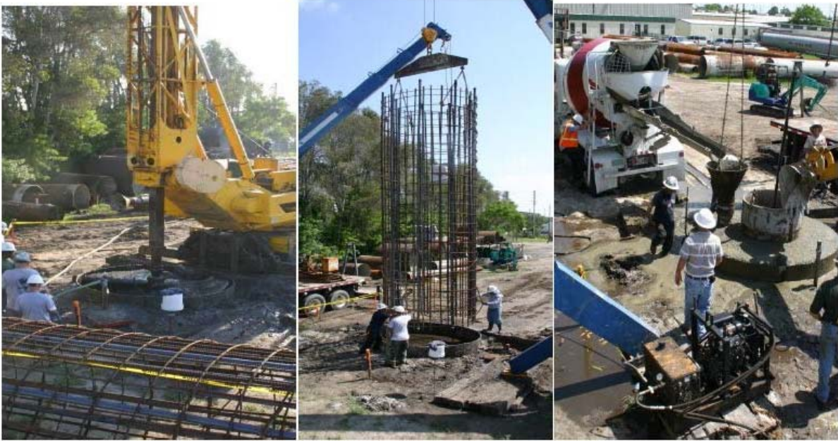
Figure 1.1 Drilled shaft construction. excavation (left) reinforcement placement (middle), concreting (right)
