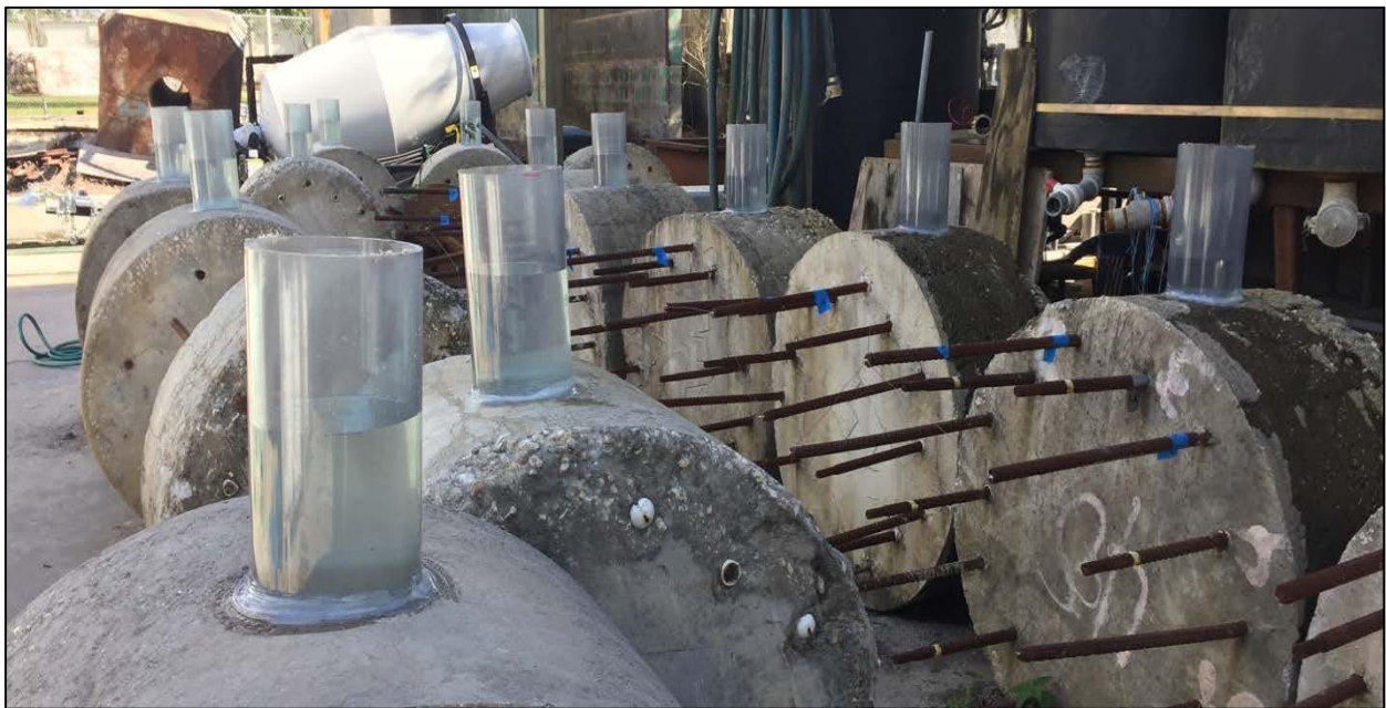
Figure 3.12 Tanks installed on shafts
