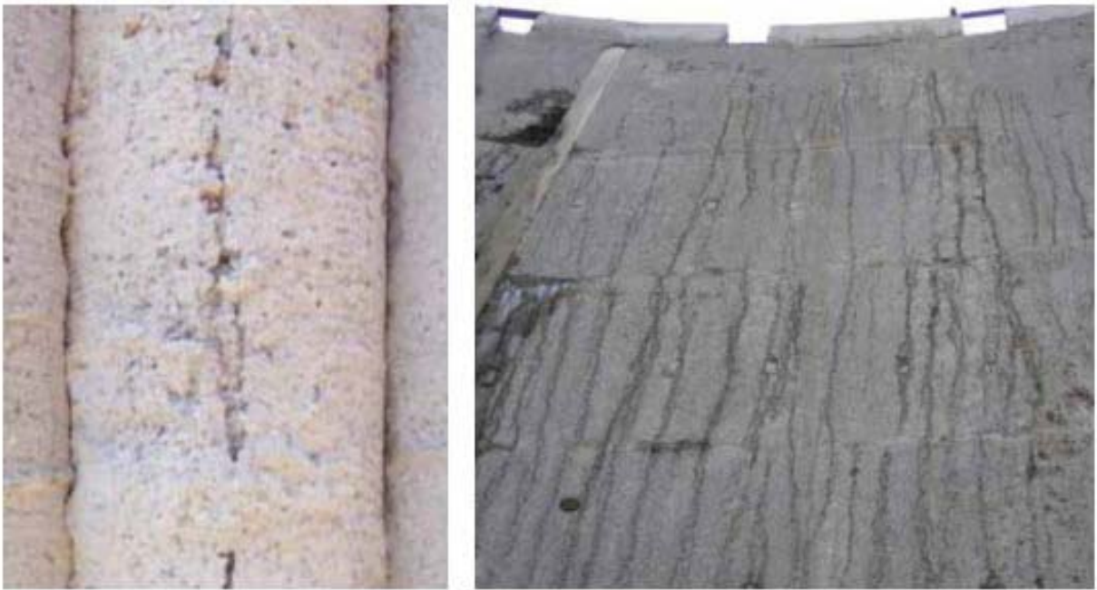
Figure 2.4 Channeling (DFI, 2016)
