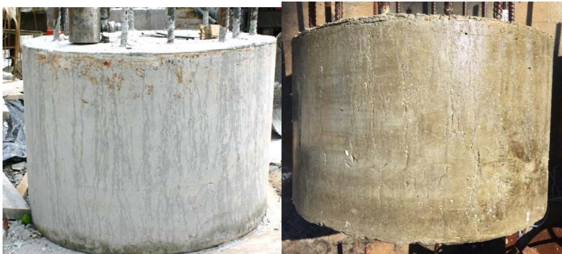
Figure 2.24 Shaft 18: f'c 4753 psi; drilled shaft mix, water cast, smooth minor channeling
