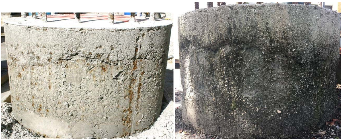
Figure 2.30 Shaft 24: self consolidating concrete, 40 second bentonite slurry, rough disintegrating
