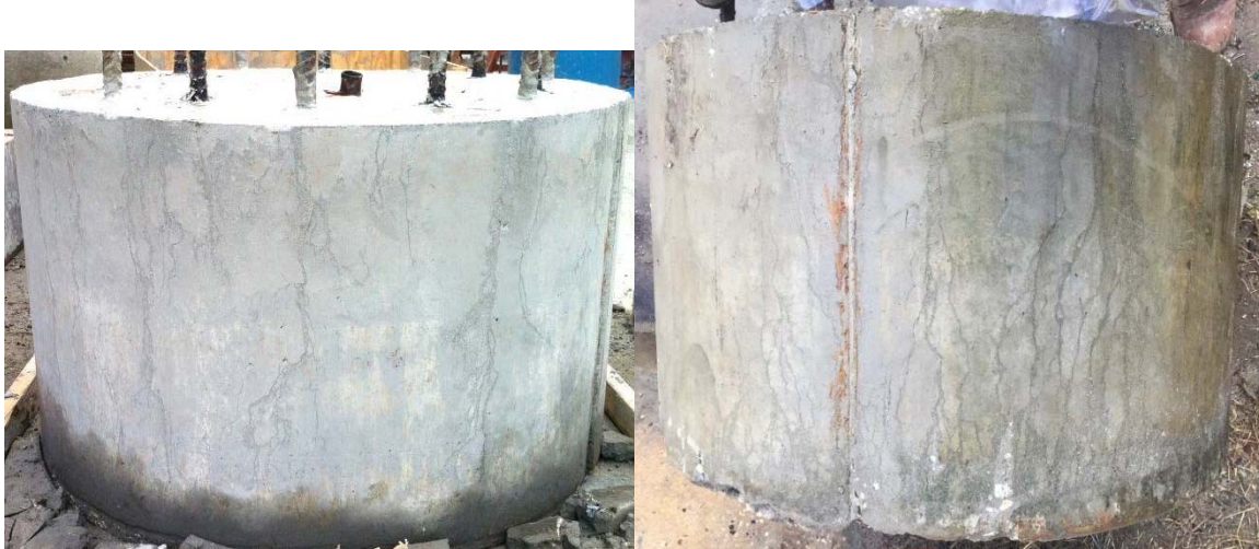
Figure 2.28 Shaft 22: f'c 4100 psi; drilled shaft mix, water cast, smooth minor channeling
