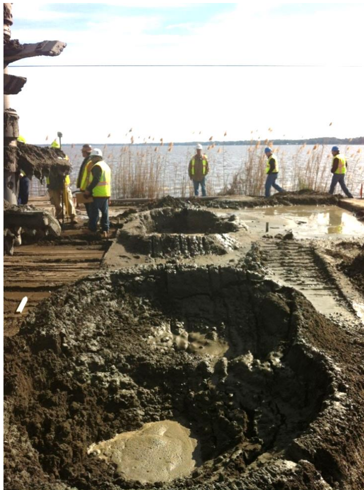
Figure 4.18. Soil mixing spoils around twin auger soil mixed demonstration elements.
