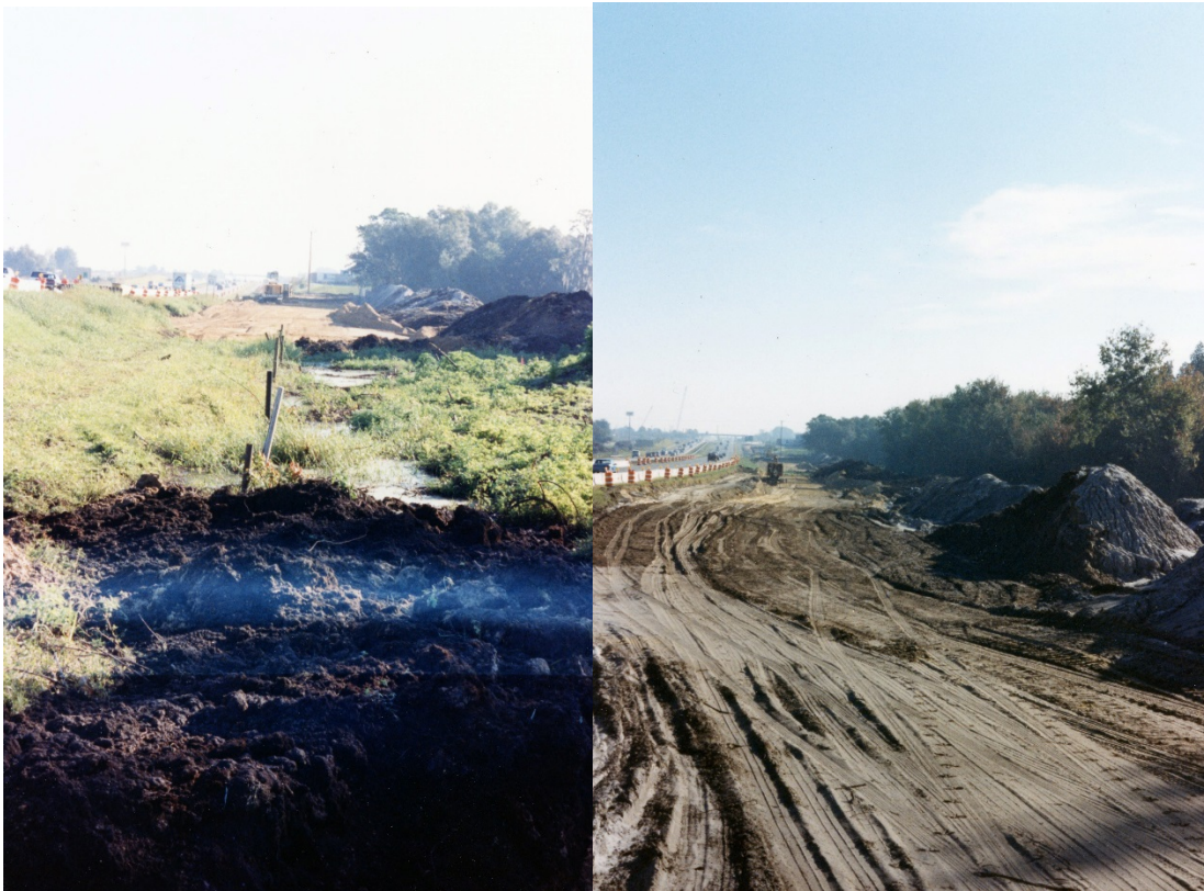
Figure 1.2. Before and after organic soil replacement on I-4.
