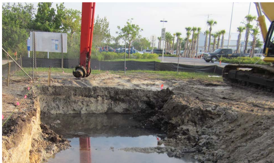
Figure 2.2. Tilling type mixing tool for DSM mass stabilization, (Baker, 2015).
