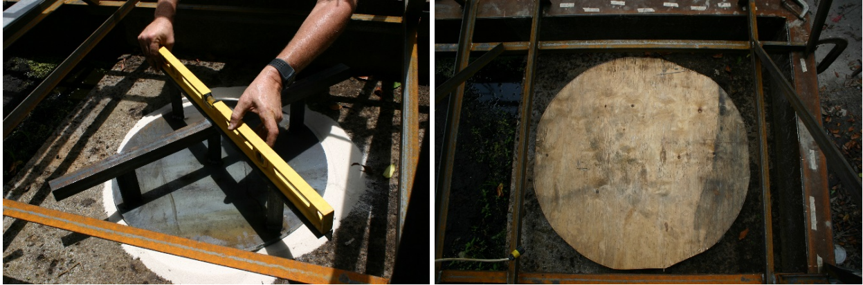
Figure 3.23. Closer look at bearing plate set up (sand, wood, then steel plate).
