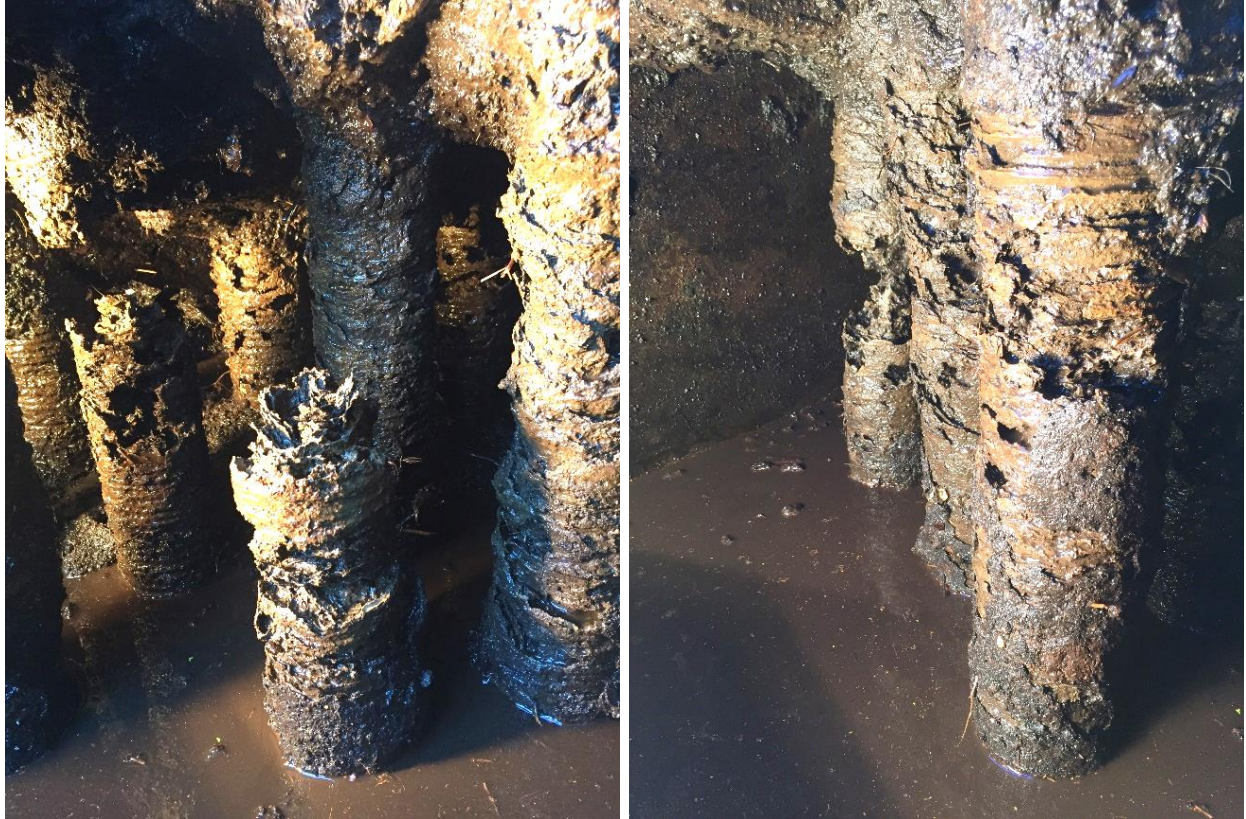
Figure 3.31. A column that was unable to be salvaged (left), versus columns that were able to be salvaged and tested (right).
