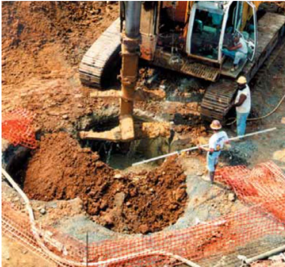
Figure 2.1. Wet soil mixing equipment (Garbin and Mann, 2012).
