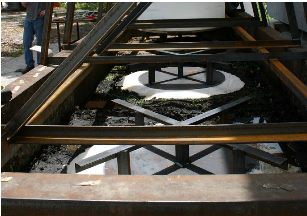
Figure 3.22. Bearing plate assembly.
