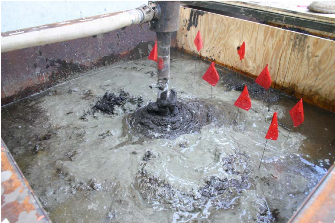
Figure 3.14. Wet mixing process up close.
