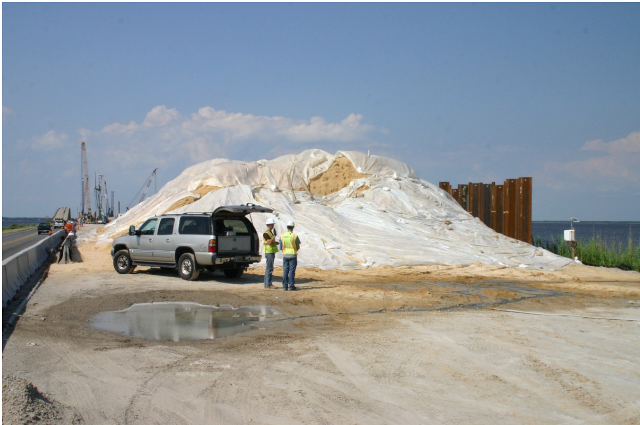
Figure 4.24. Surcharge / embankment load fully in place on test section (approx. 19ft).
