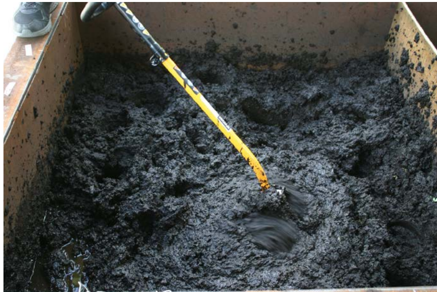
Figure 3.16. Initial breakup of the saturated organic soil prior to adding cement.
