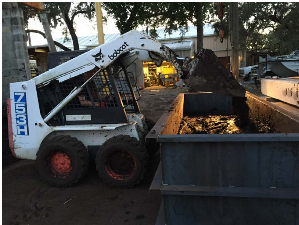
Figure 3.4. Transfer of the soil to the test bed.
