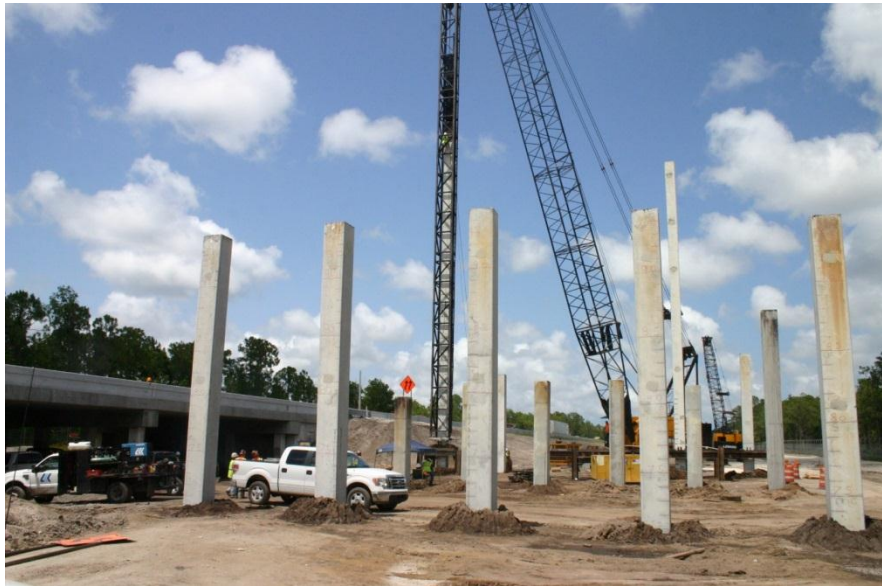
Figure 1.1 Deep foundation construction.
