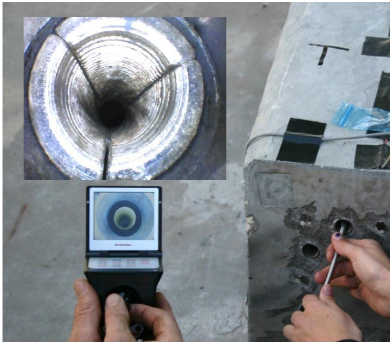
Figure 3.10 Inspection of ducts using borescope.
