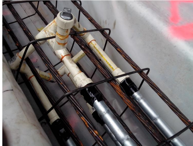
Figure 2.24 Grouting manifold.
