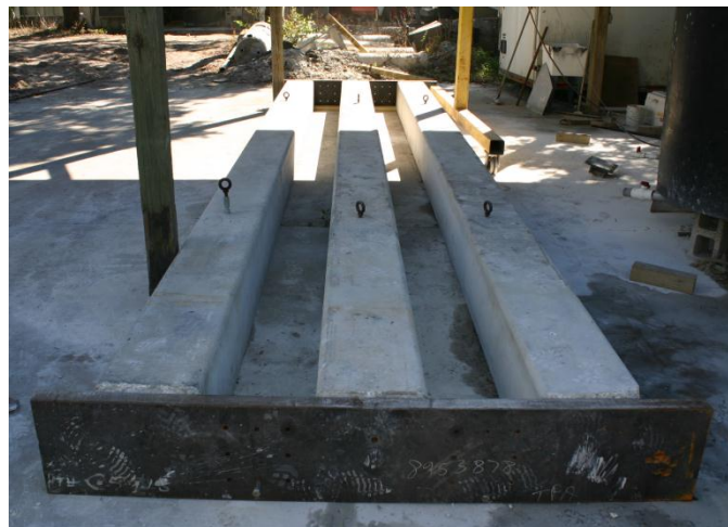
Figure 3.2 Casting bed for test piles.
