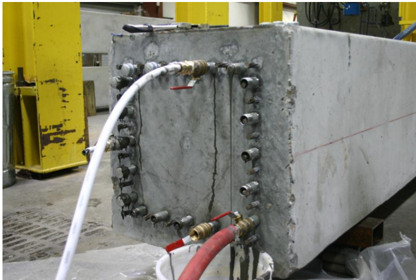
Figure 4.10 Grouting post-tensioned strand ducts.
