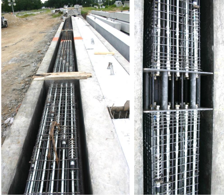
Figure 4.5 Fully stressed bed (left) and splicing header connection (right).
