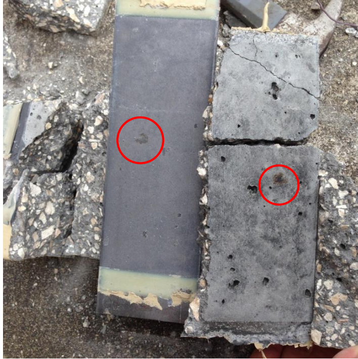
Figure E.5 Corrosion spots on the steel-concrete interface of specimen L6
