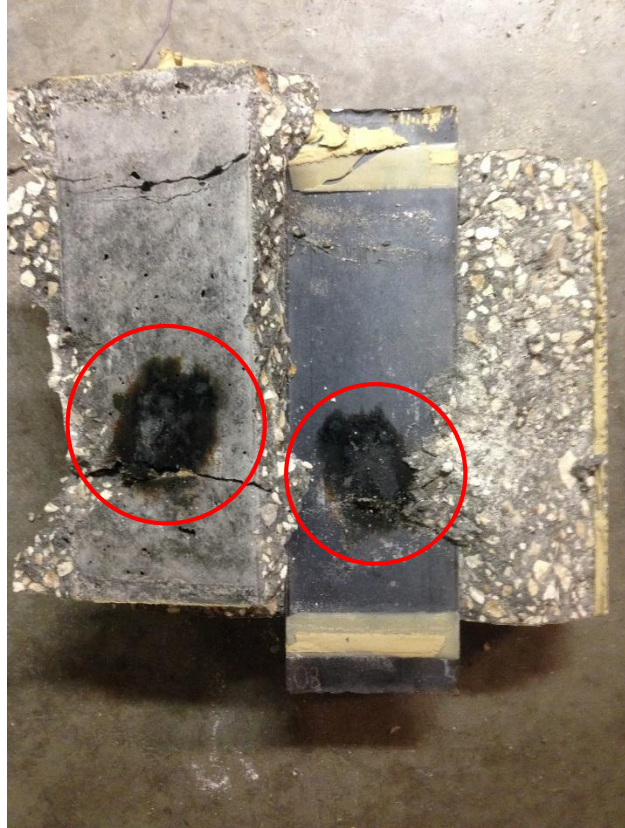
Figure E.11 Corrosion spots on the steel-concrete interface of specimen S8
