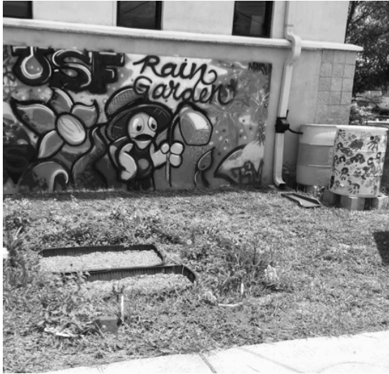
Figure 3.1 Bioretention Cells at the Corporation to Develop Communities, Audrey L. Spotford Youth and Family Center (Tampa, FL)
