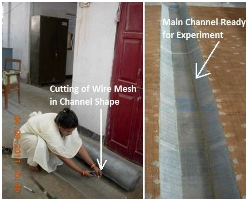
Fig. 3.10 Construction of mesh roughened main channel
