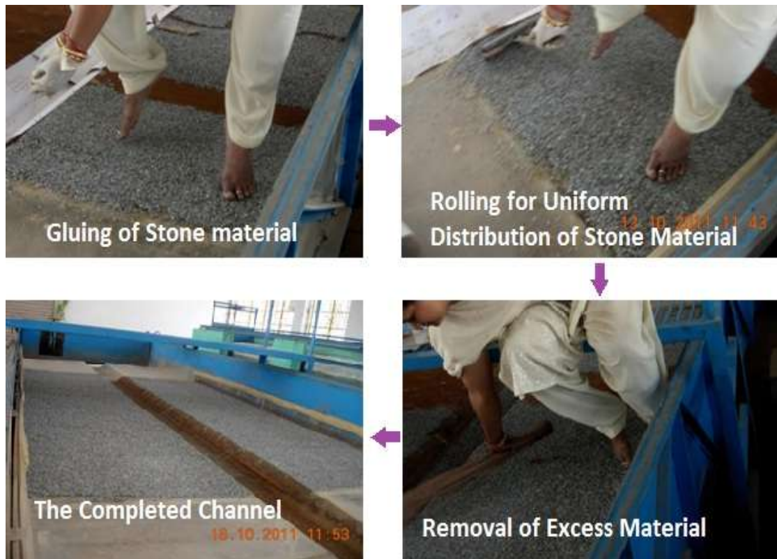
Fig. 3.17 Construction of Roughness-II
