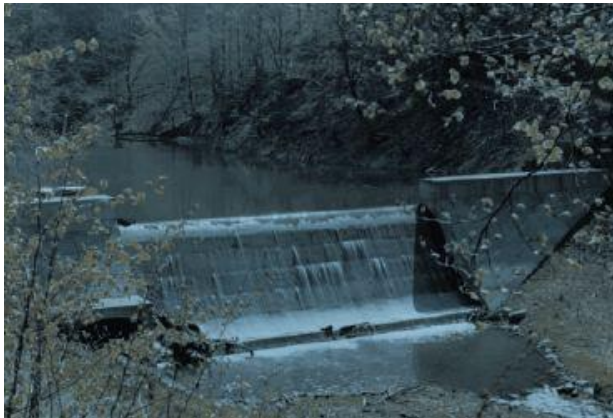
Figure 4.9(a): Concrete weir
