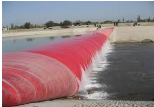
Figure 4.9(b): Inflated weir
