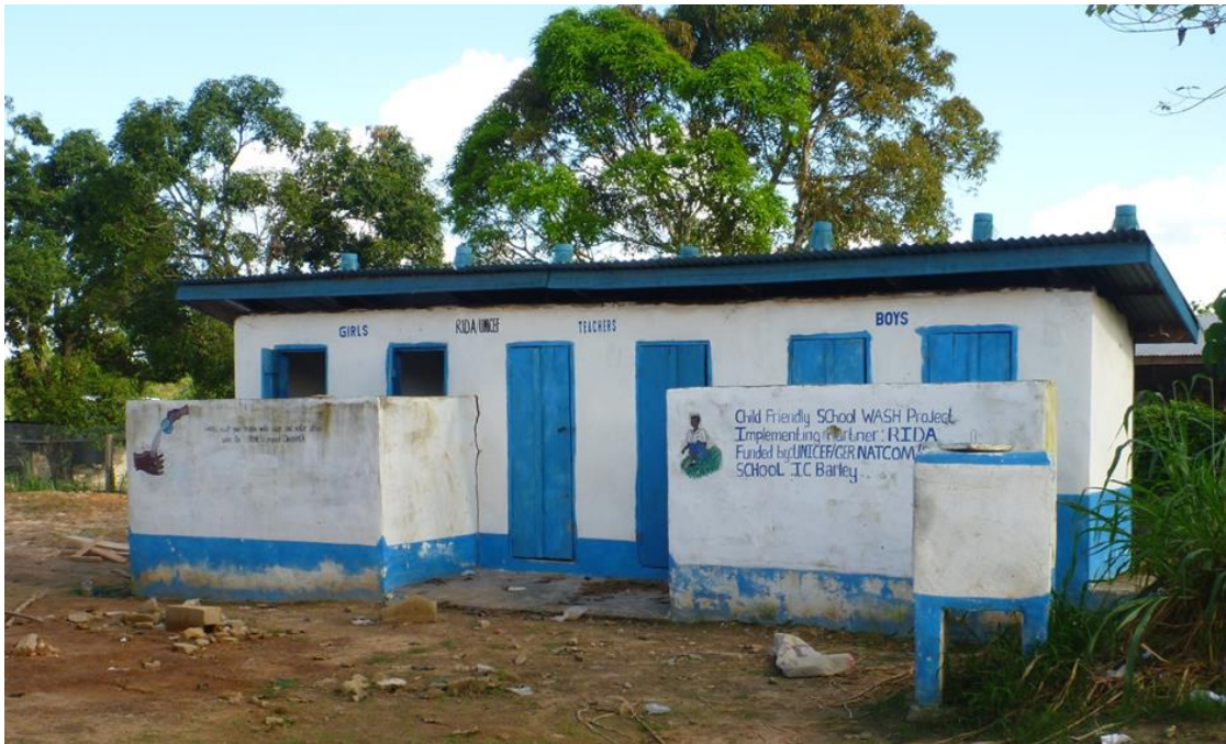
Figure 6 School VIP latrine block with six stalls.
