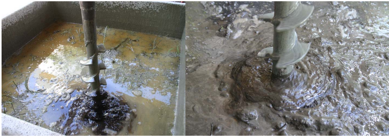
Figure 4.16 Test column being wet mixed (left); close up (right).
