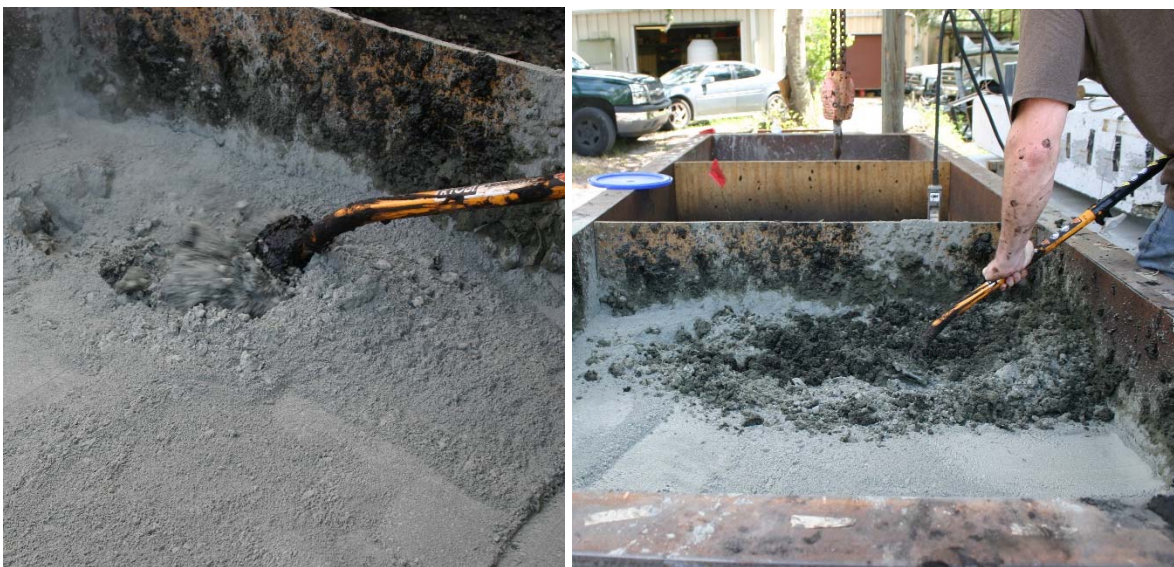
Figure 4.30 Dry mixing progression, part 1 of 2.
