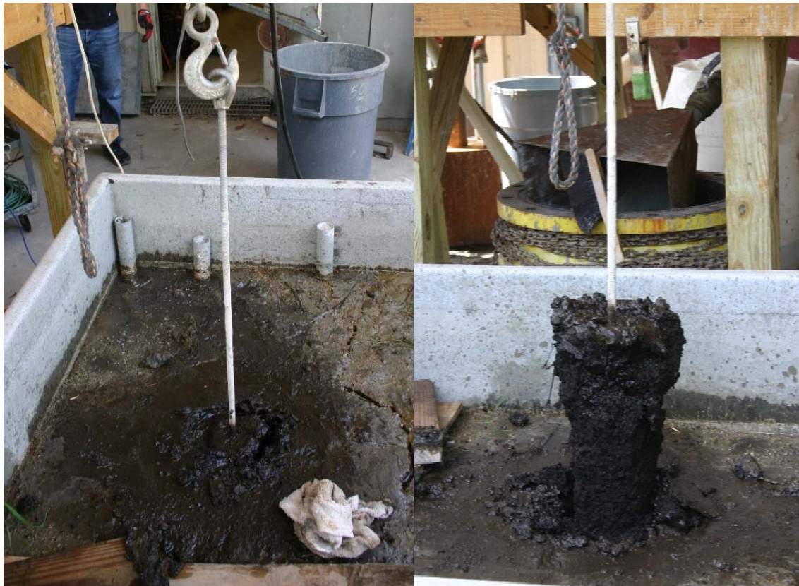
Figure 4.17 Wet mixed column being removed from soil after 28 days.
