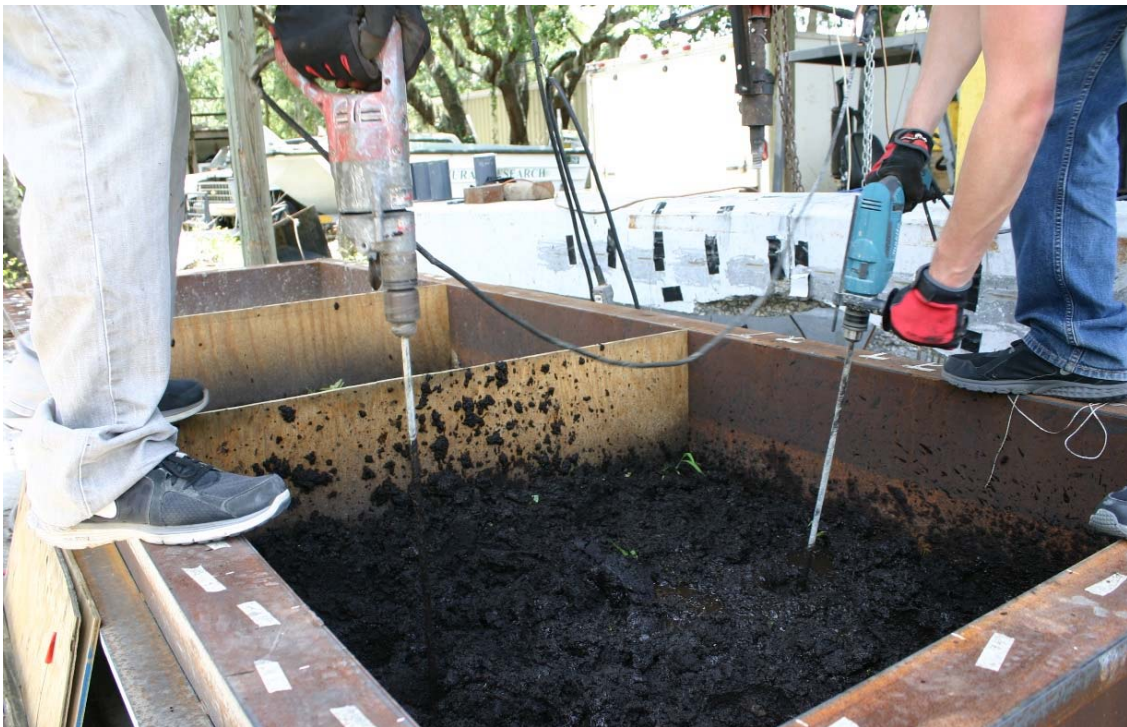
Figure 4.27 Two mixing paddles breaking up soil.
