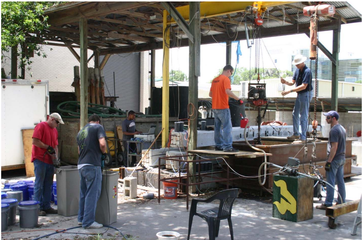
Figure 4.23 Wet mixing in steel bed overview.
