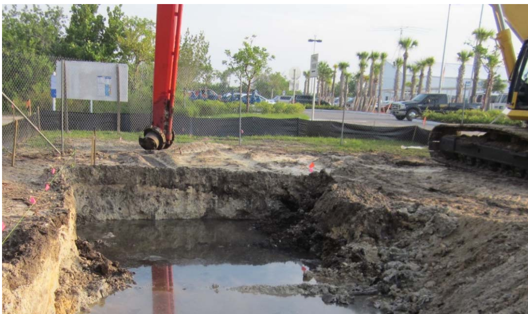
Figure 2.2 Tilling type mixing tool for DSM mass stabilization (2 to 3 ft diameter and 5 ft wide).
