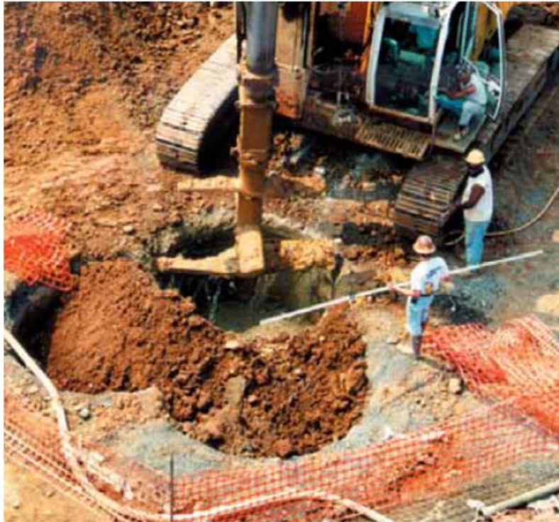
Figure 2.1 Wet soil mixing equipment (courtesy of Hayward Baker).
