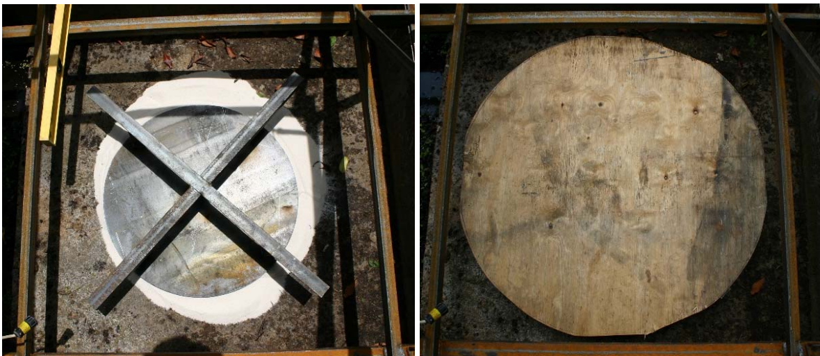
Figure 4.34 Bearing plate assembly with plywood.
