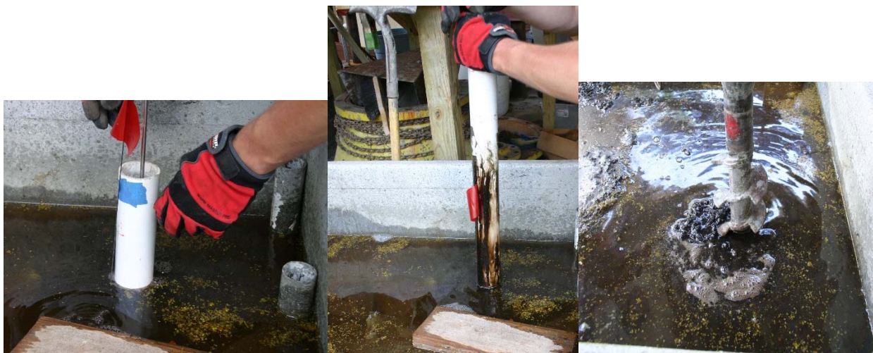
Figure 4.20 Testing of dry mixing concept.
