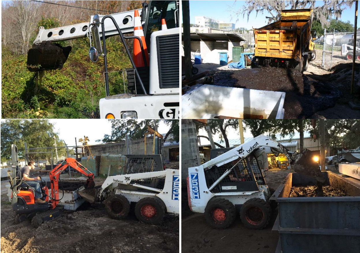
Figure 4.4 Excavation and delivery of organic soil to bed.
