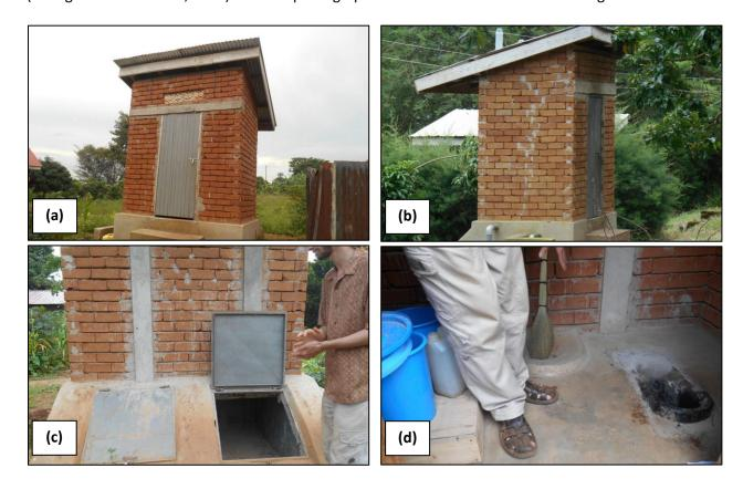
Figure 4: Demonstration UDDTs installed in primary schools in Kalisizo, Uganda (all photographs taken by Debra Trimmer). (a) External front view; (b) external side view; (c) external rear view, showing two fecal collection vaults; (d) internal view, showing the urine diversion device
