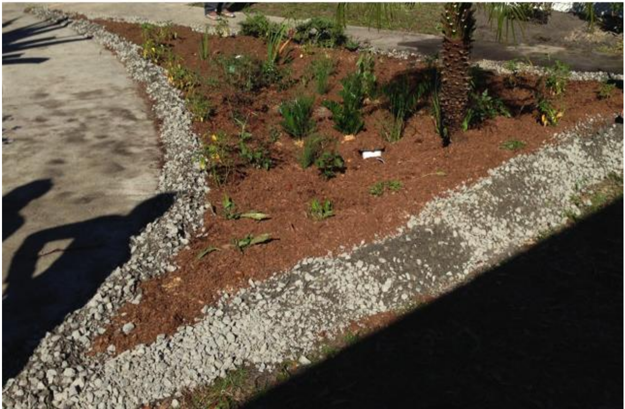
Figure 14: Bioretention BR 8 pre-construction (top) and post-construction (bottom)
