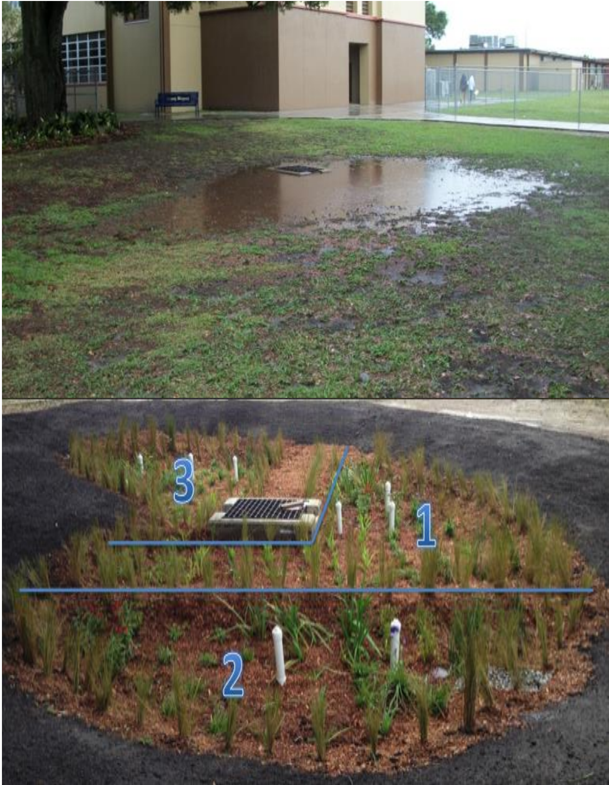
Figure 11: Bioretention BR 1, BR 2, BR 3 pre-construction (top) and post-construction (bottom)
