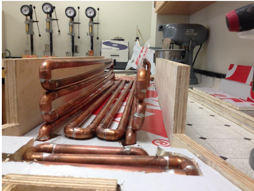
Figure A-6: Copper Piping Throughout RCF Formwork
