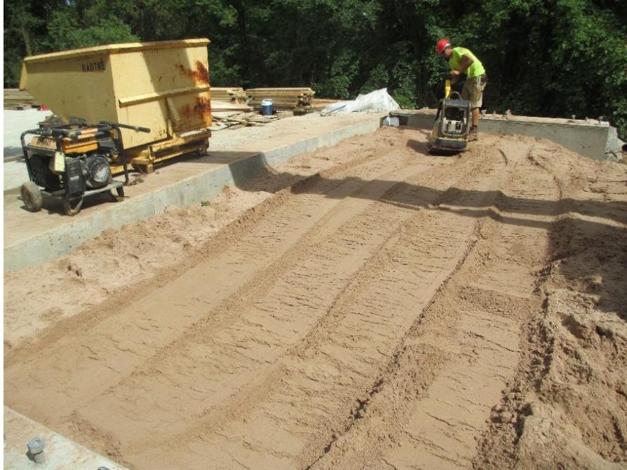
Figure 102. Compaction of backfill at Schwartz Road Bridge
