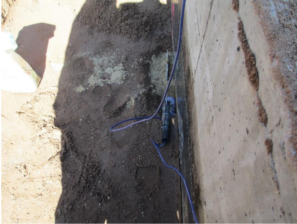
Figure 126. Lateral EPC installation at Hobbles Creek Bridge
