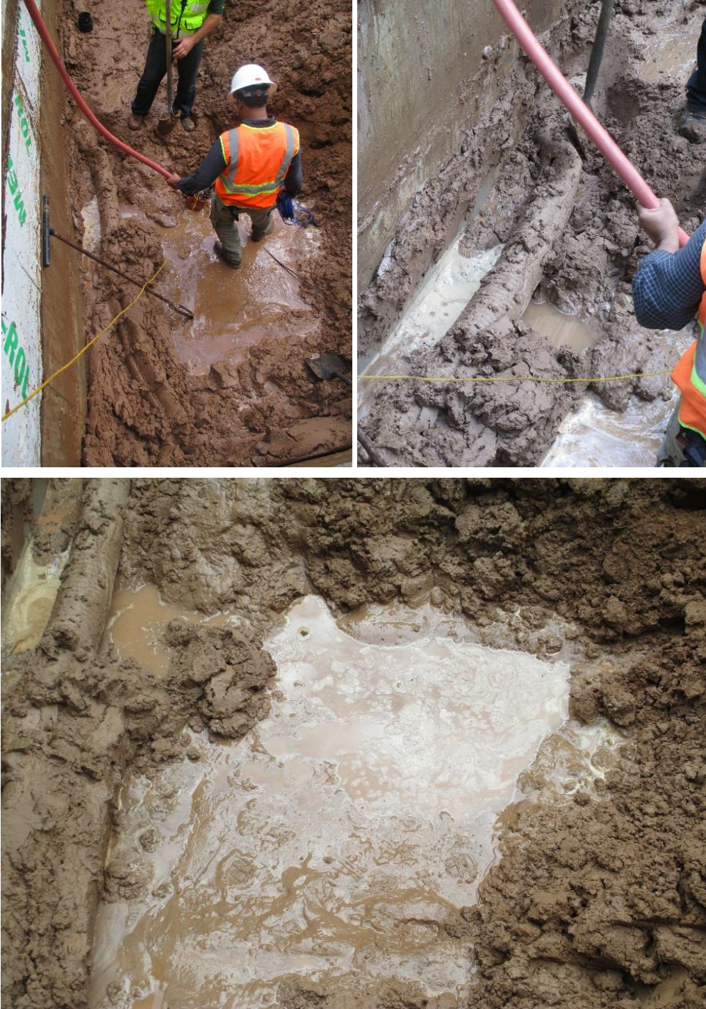
Figure 101. Bottom of the excavation near the drain tile on the south abutment after pumping out the ponded water
