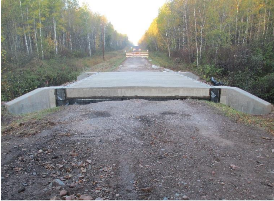
Figure 116. Hobbles Creek Bridge west abutment before backfilling
