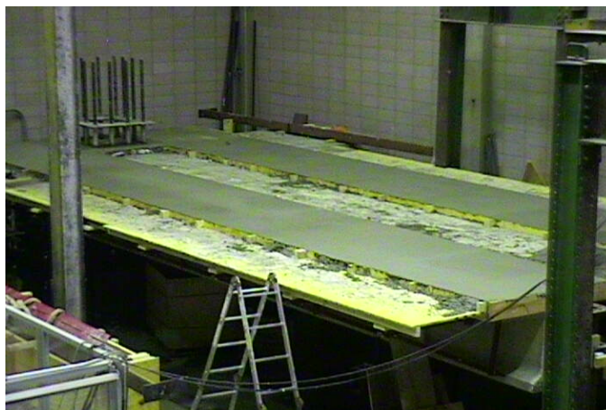
Figure 3.21: Completed cap and deck concrete pour
