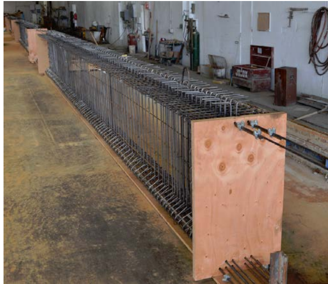
Figure 3.16: Girder strand layout and rebar cage
