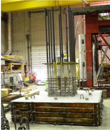
Figure 3.13: Footing and Column pour
