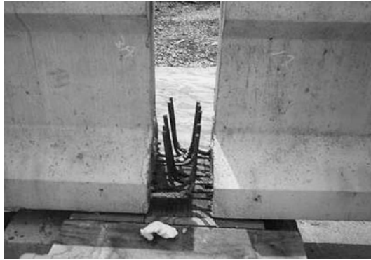
Figure 2.27: Bent reinforcing bar connection (NCHRP, 2004)
