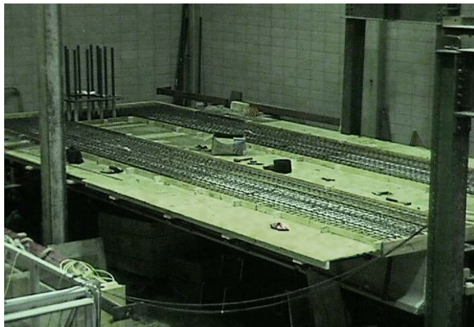
Figure 3.20: Deck formwork and rebar
