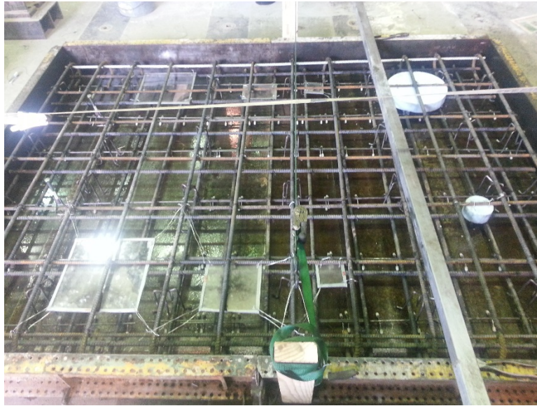
Figure 5.7. Photo of formwork and rebar cage for mock-up bridge deck containing artificial defects before casting.
