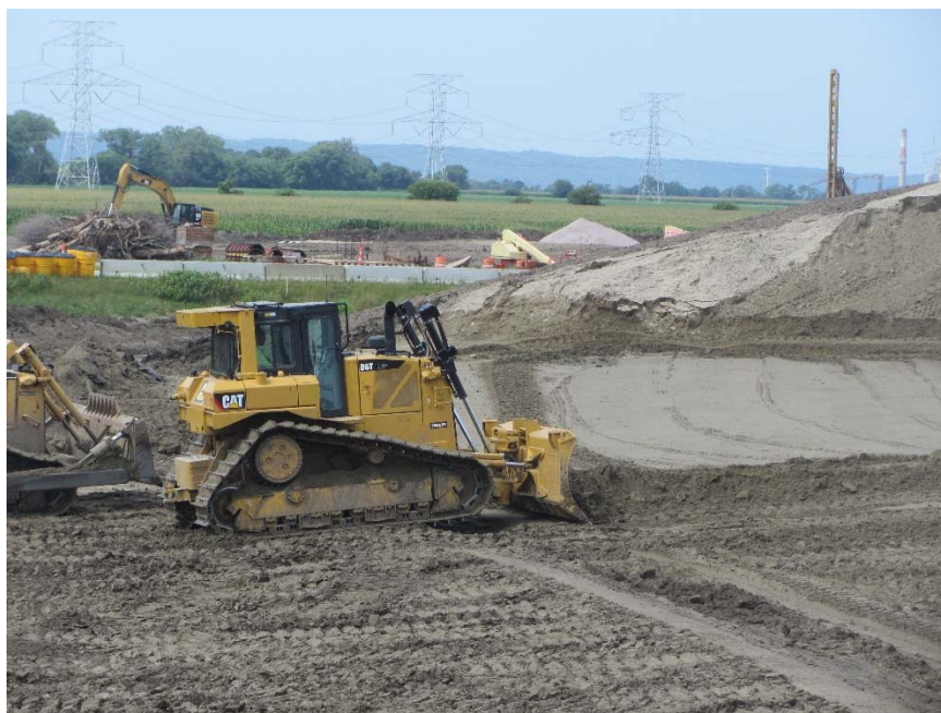
Figure 96. Caterpillar D6T dozer used to control lift thickness
