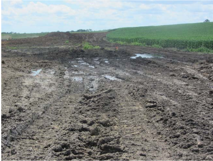
Figure 58. Seepage occurred in the construction site
