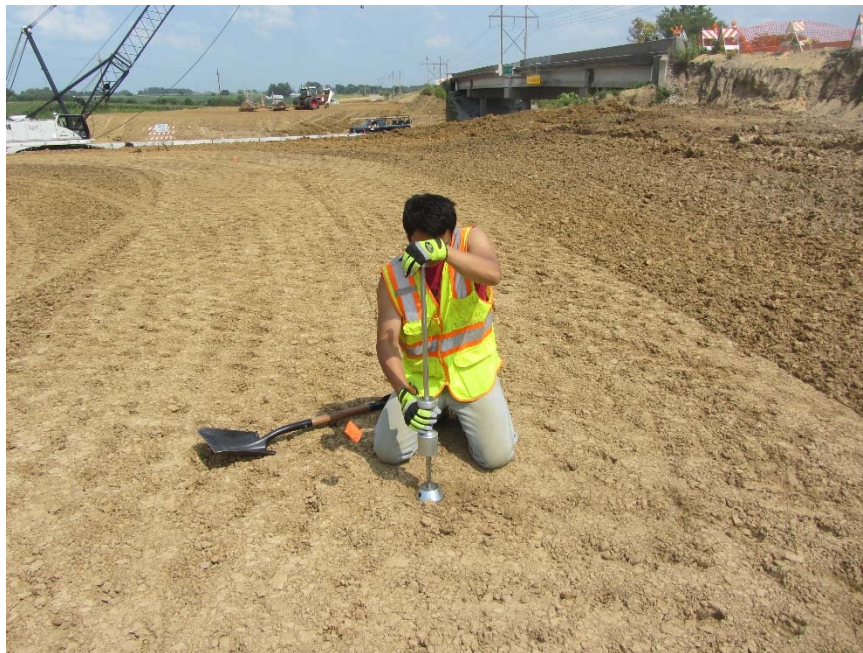
Figure 112. ISU in situ drive cylinder testing
