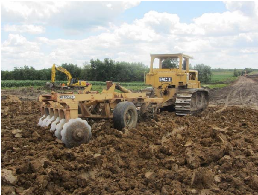
Figure 55. Disk used to dry embankment materials
