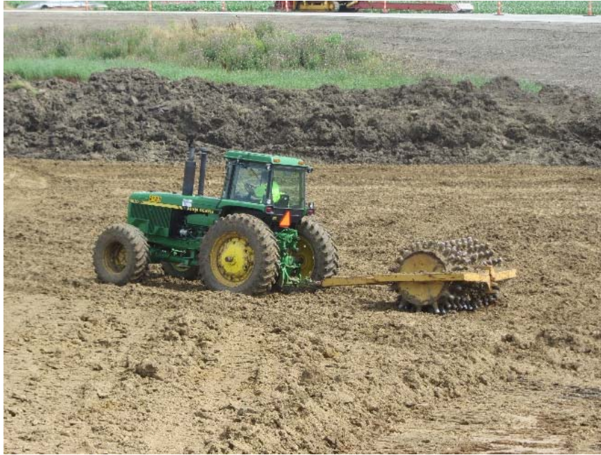
Figure 79. Sheepfoot roller used for soil compaction
