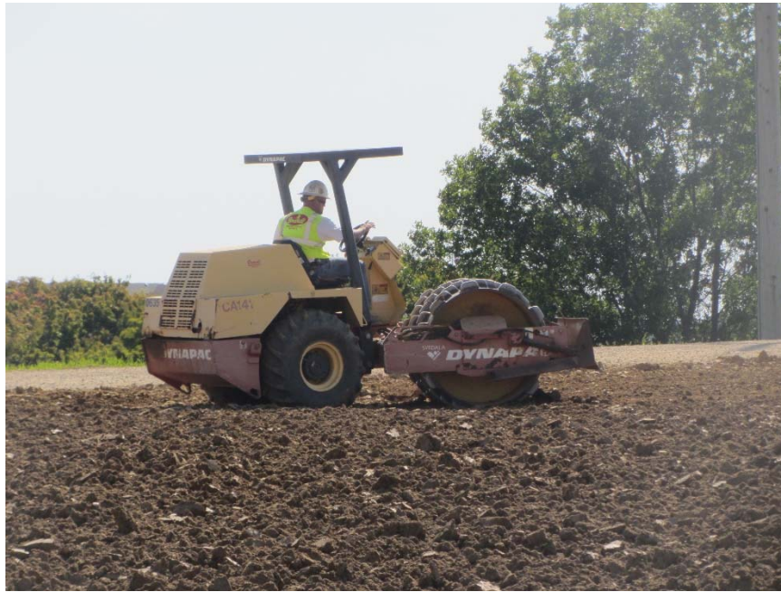
Figure 111. Dynapac pad foot roller used for soil compaction
