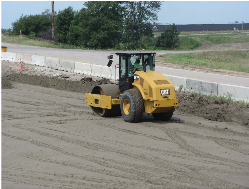
Figure 97. Caterpillar CS56B vibratory smooth drum roller used for soil compaction
