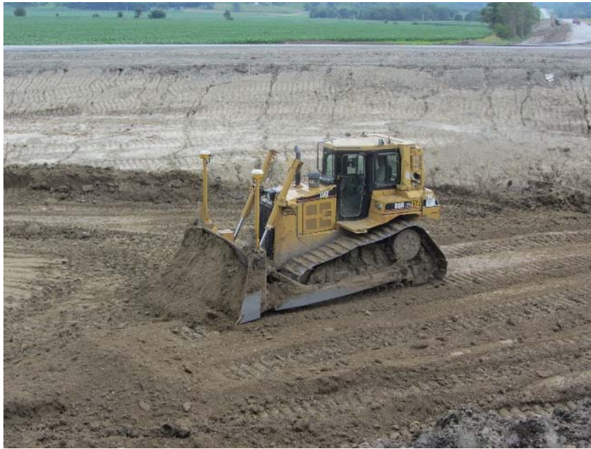
Figure 77. Caterpillar D6R dozer used to control lift thickness
