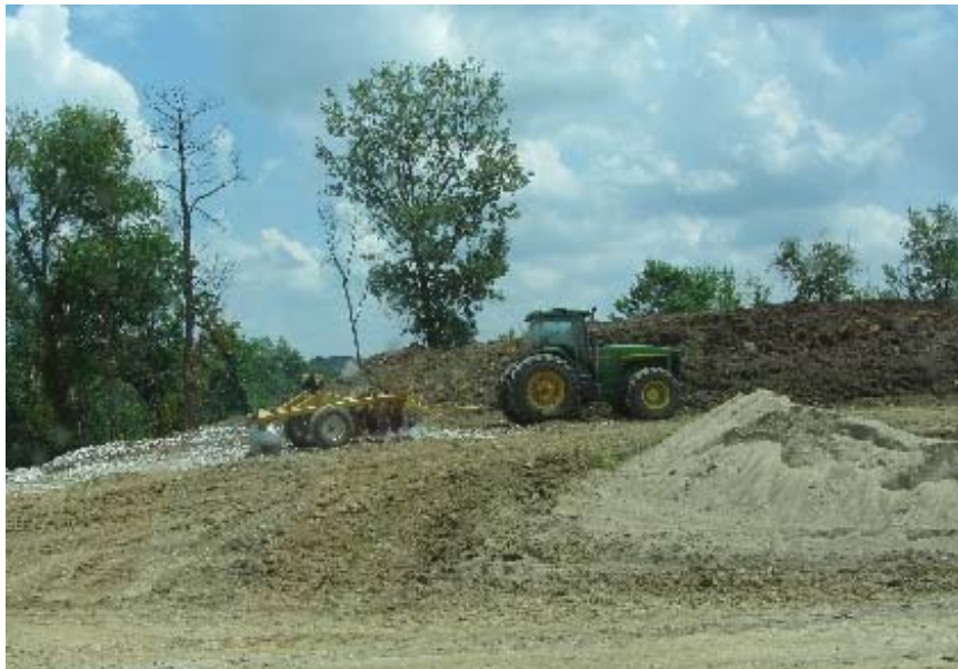
Figure 31. Disk used to dry embankment materials
