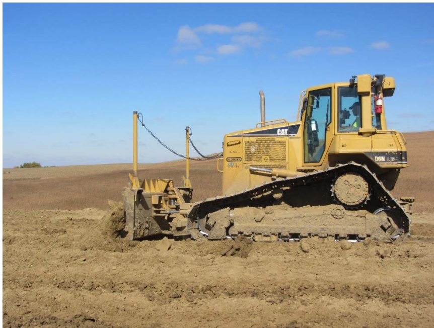
Figure 120. Caterpillar D6N dozer used to control lift thickness
