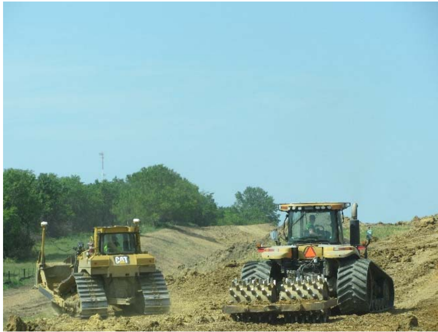
Figure 45. Sheepfoot roller used for soil compaction
