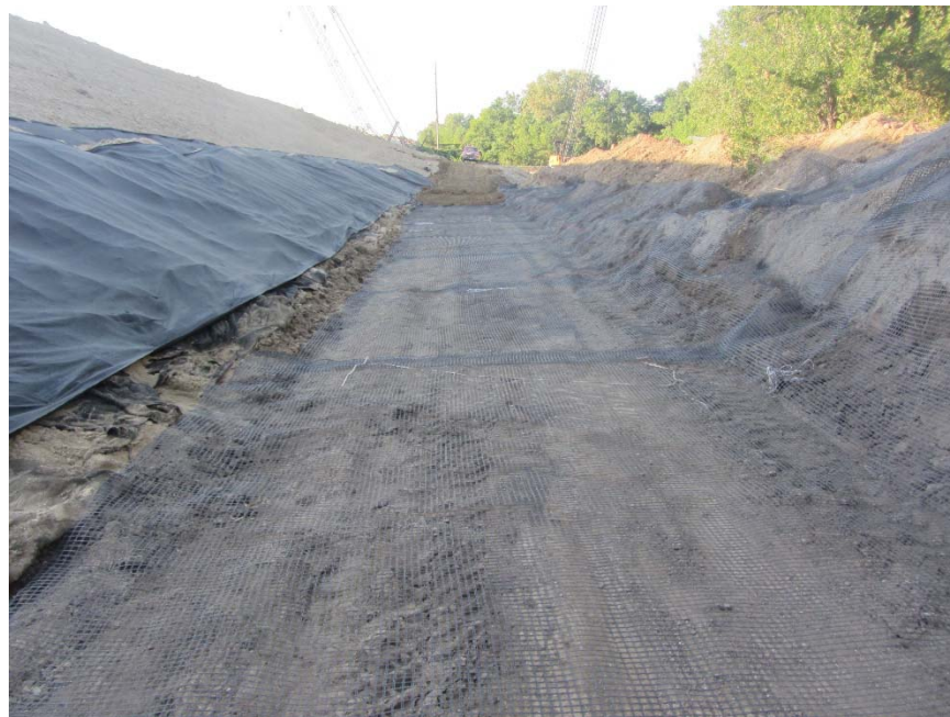
Figure 35. Geogrid placed near embankment toe
