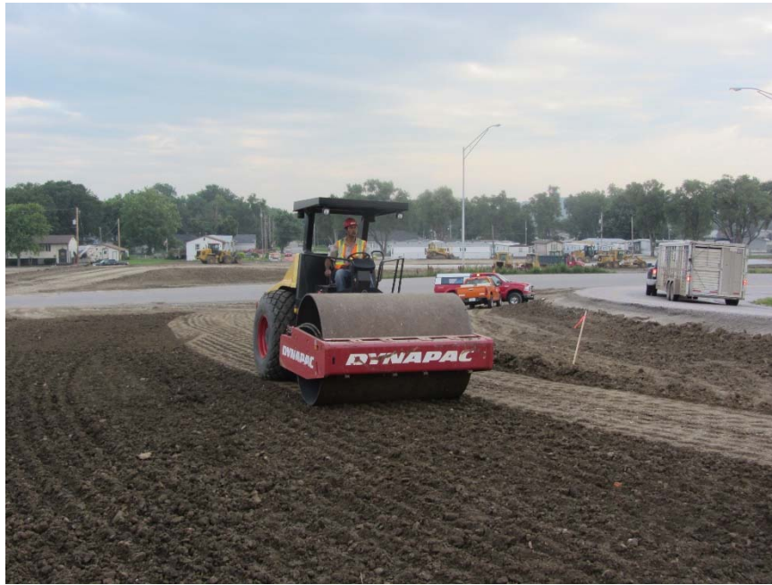
Figure 88. Dynapac CA250-II vibratory smooth drum roller used for soil compaction
