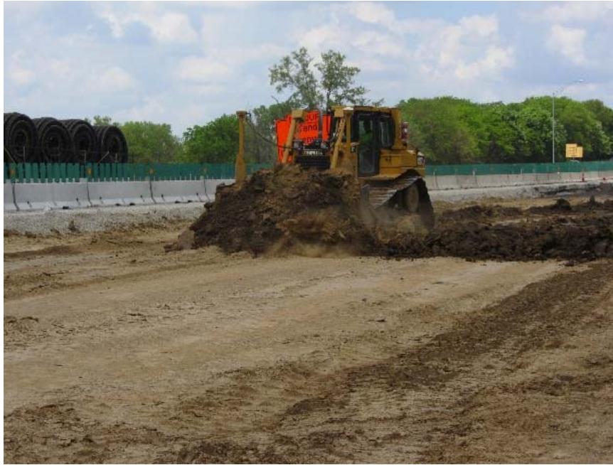
Figure 32. Caterpillar D6T Dozer used to control lift thickness
