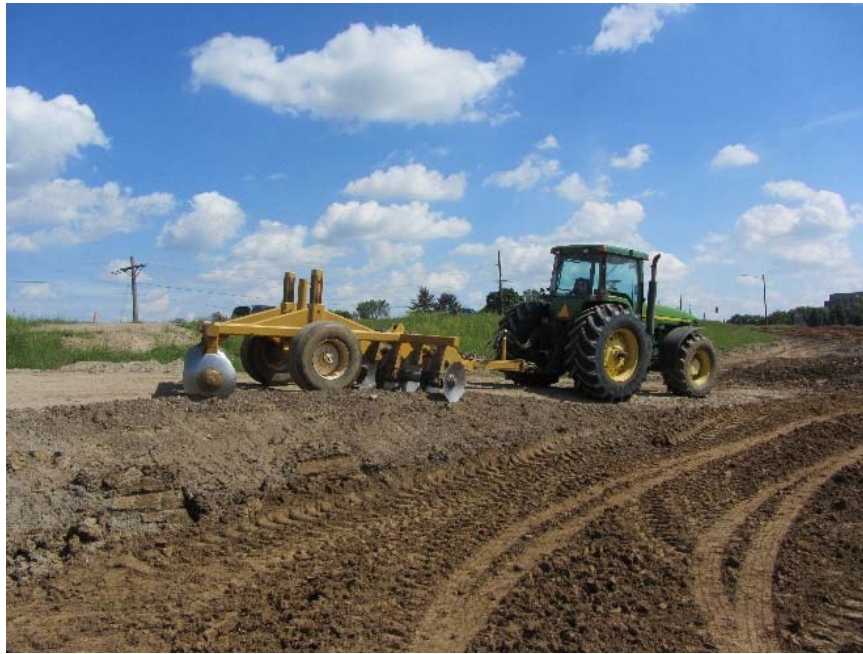
Figure 70. Disk appear on site used to dry materials
