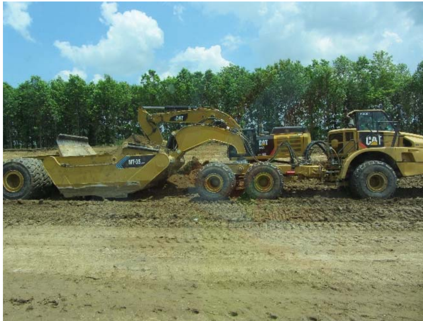
Figure 28. Caterpillar MT-35 scraper used to collect and place loose fill materials
