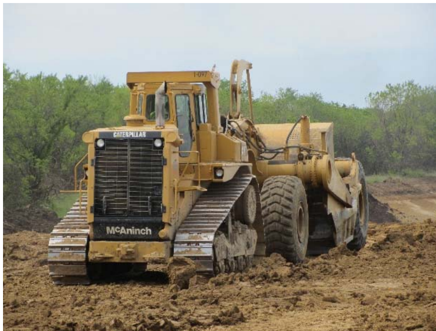
Figure 44. Caterpillar MT-35 scraper used to collect and place loose fill materials
