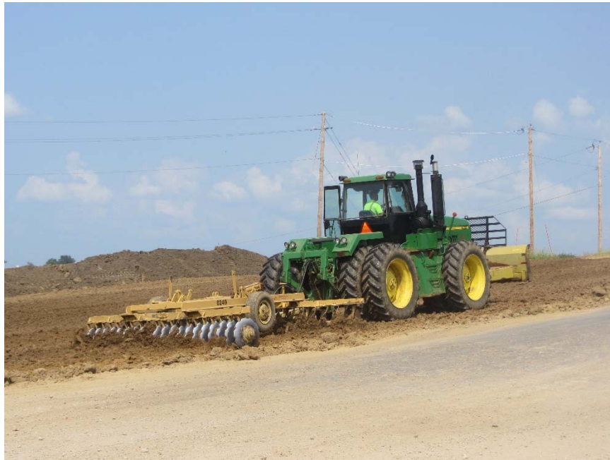
Figure 109. Disk used to dry embankment materials
