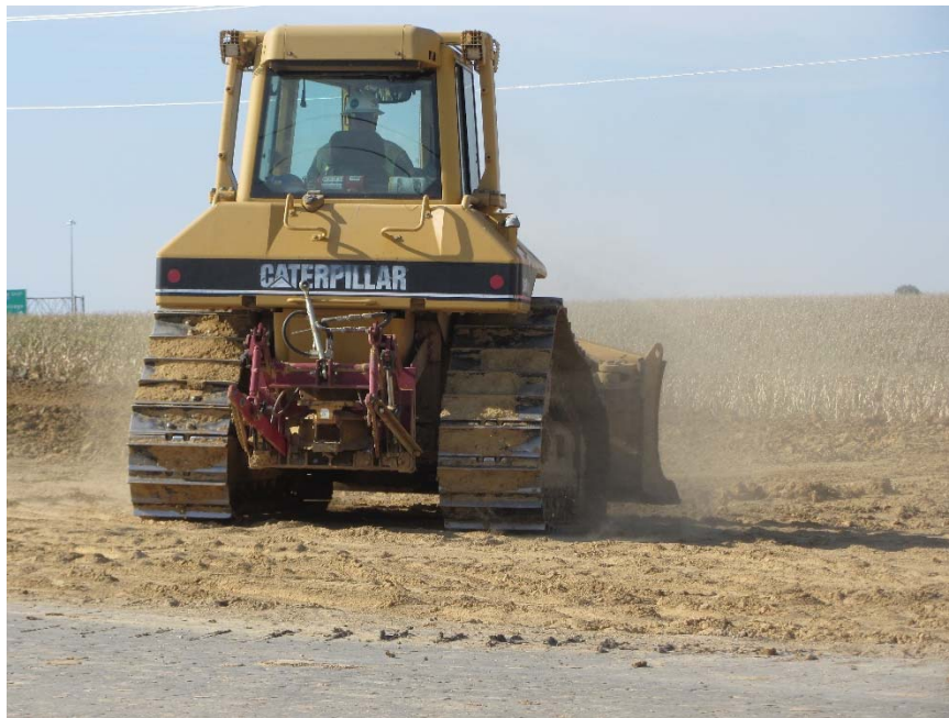
Figure 108. Caterpillar dozer used to control lift thickness
