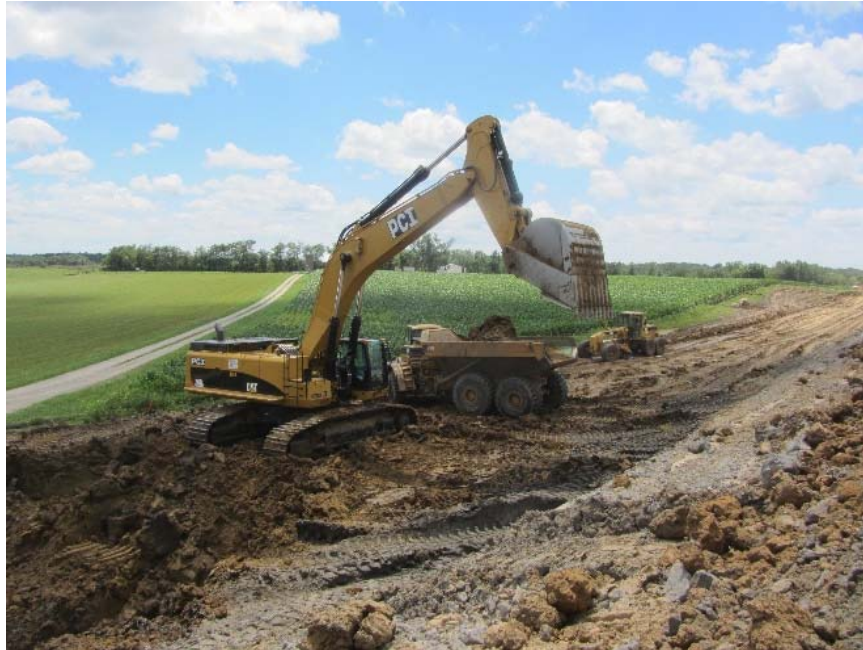
Figure 53. Caterpillar 390D excavated materials from borrow source
