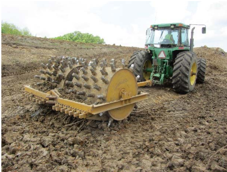
Figure 33. Sheepfoot roller used for soil compaction
