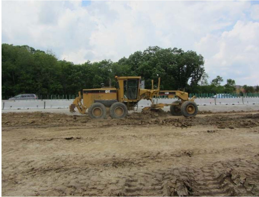
Figure 30. Caterpillar 143H motor grader used to level the embankment surface
