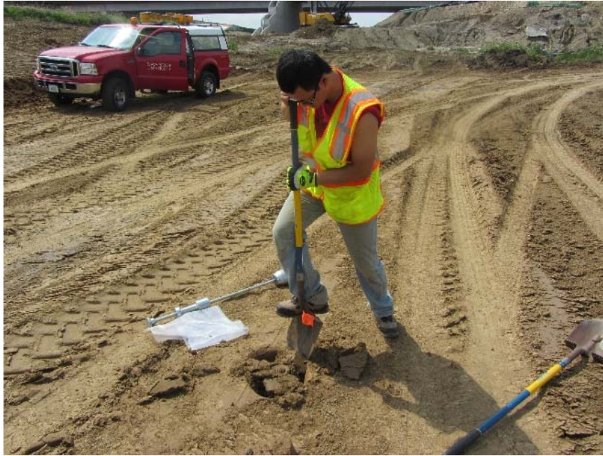
Figure 81. ISU in situ drive cylinder test
