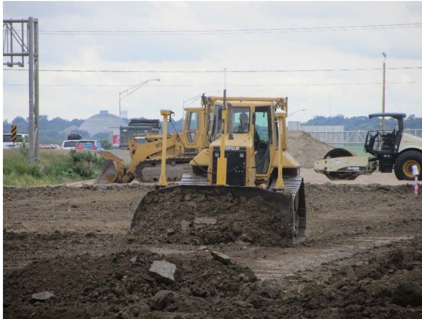
Figure 86. Caterpillar dozer used to control lift thickness
