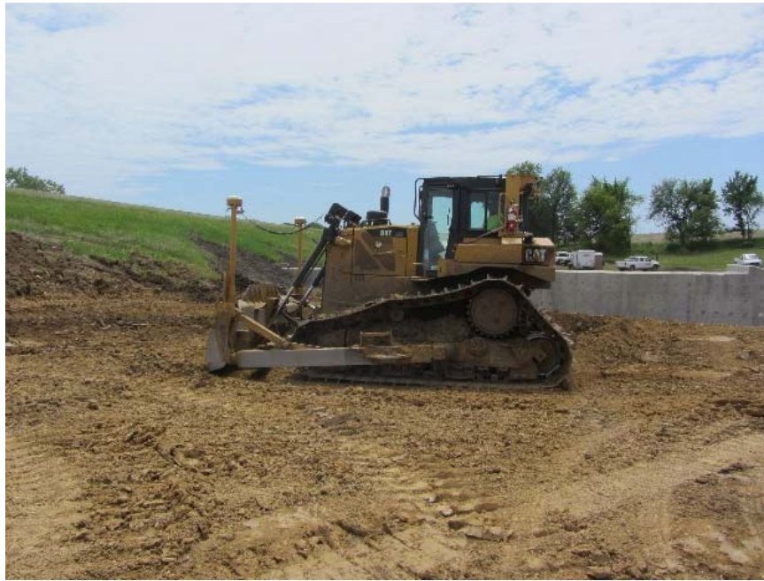
Figure 43. Caterpillar D6T Dozer used to control lift thickness
