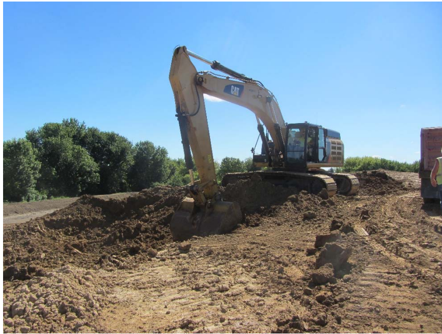
Figure 107. Caterpillar 349E excavate materials from borrow source
