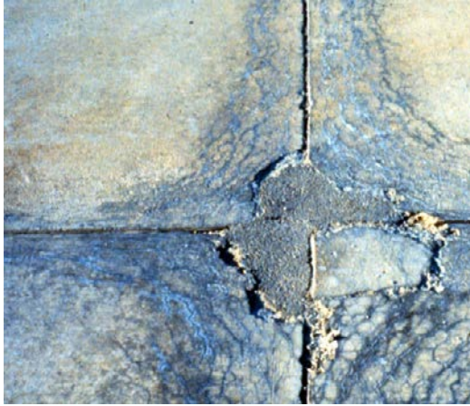
(a) D-cracking at a Joint Intersection
