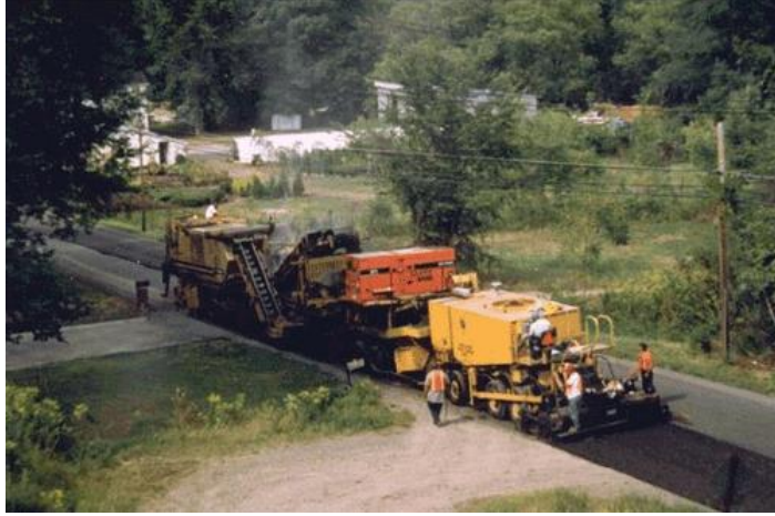
Figure 9 Cold In-Place Recycling (CIR or CIPR) (Source: FHWA)
