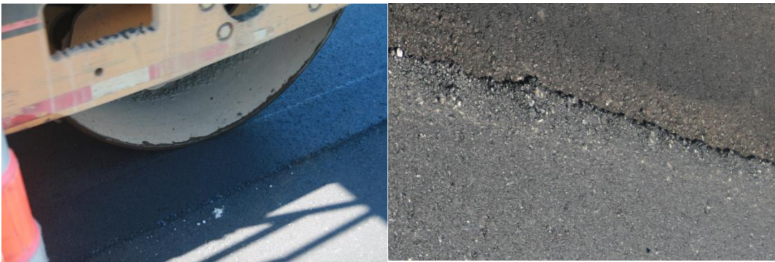
Figure 15 Butt joint construction with hot pinch (pictured on US-61)
