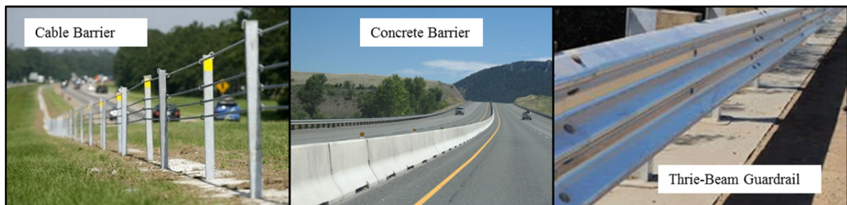
Figure 27. Median Barrier Treatment Options Used on Michigan Freeways
