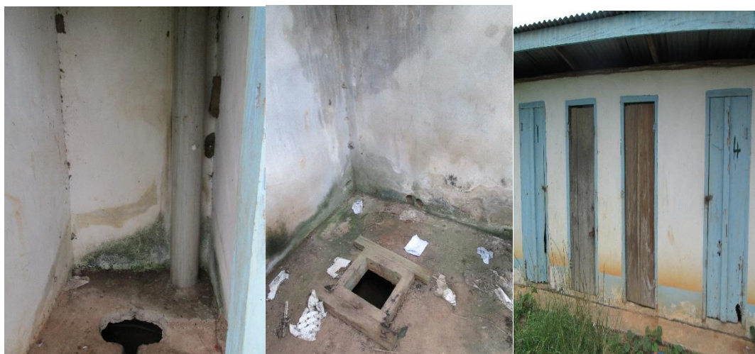
Figure 16 ULICA Mission School VIP Latrine (left), Traditional Latrine (middle), and Latrine Superstructure (right)
