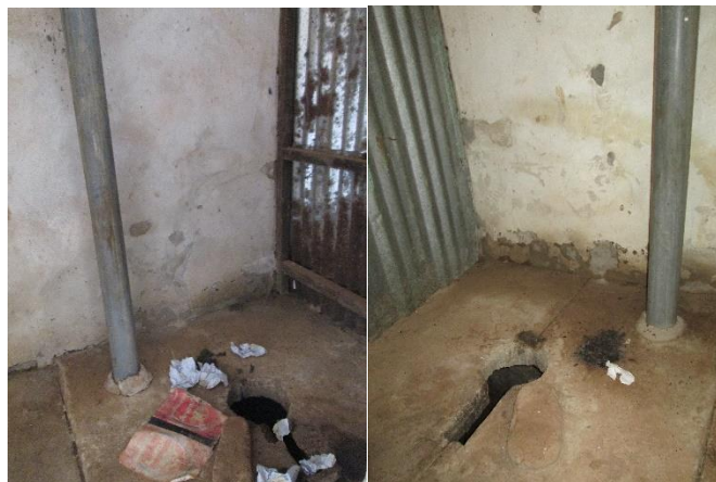
Figure 17 Red Cross School Boys' Latrine (left) and Girls' Latrine (right)
