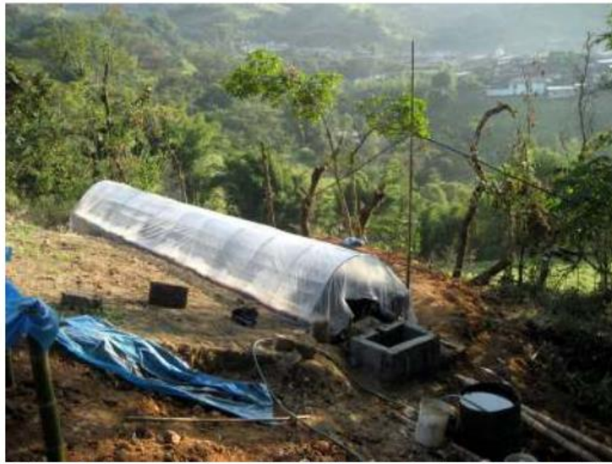
Figure 5.8 – A common tubular digester configuration with a clear plastic cover used in South America (Galvin, 2013).
