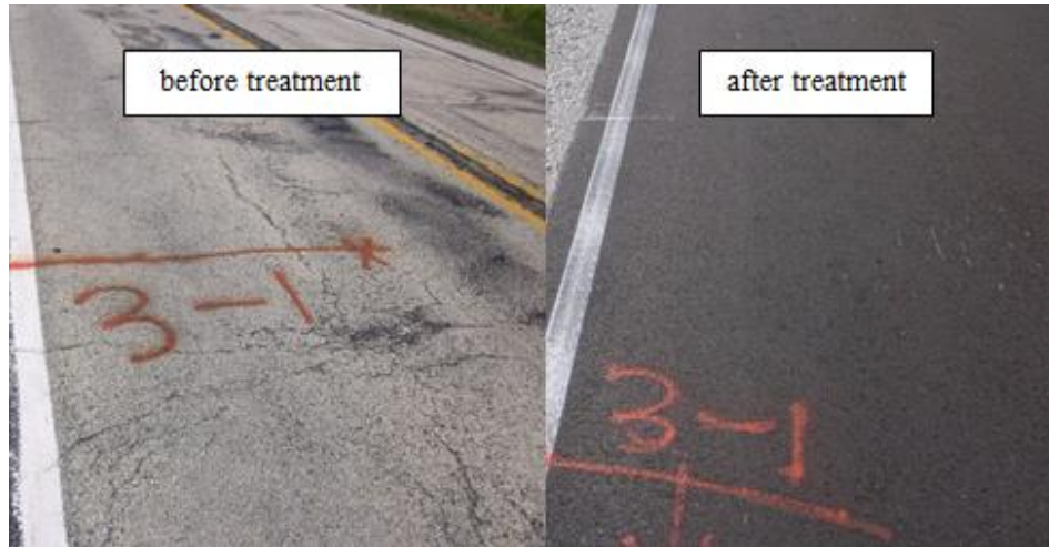
Figure 3.2. Comparison Between Surface Conditions Before and After Treatment
