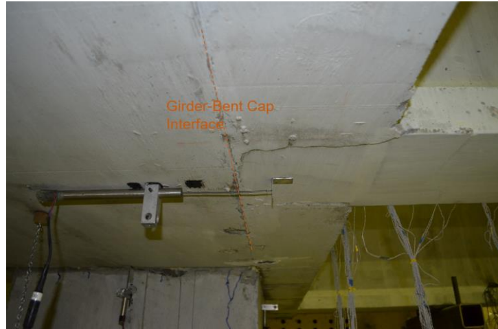
Figure 4-19 Location of LVDT on Girder-to-cap interface
