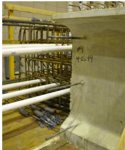
Figure 4-2 Dowel Bars Inserted through the Web of Girder
