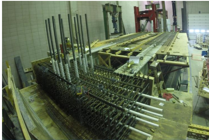
Figure 4-4 Reinforcement Cage for Bent Cap and Deck Reinforcing Steel
