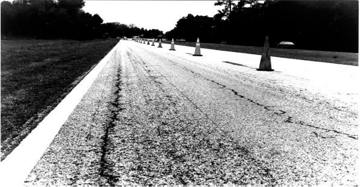
Figure 2-10 Lane exhibiting surface initiated top-down cracking in both wheelpaths (Myers et al., 2000)
