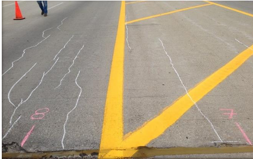
Figure 5. Longitudinal cracks at middle of deck top
