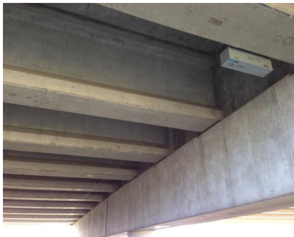
Figure 18. Vibrating wire long-range displacement meter
