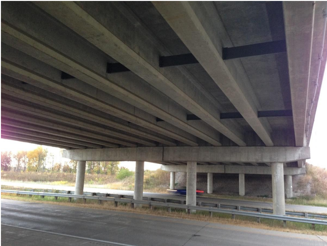
Figure 4. Bottom view of the bridge
