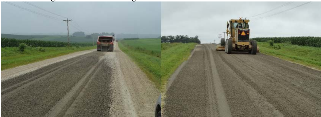
Figure 43. Construction in Goodhue County
