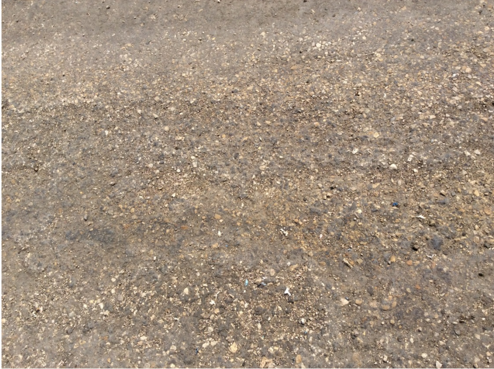
Figure 10. Close-up shot of TOSS LS CL6 2013 Section
