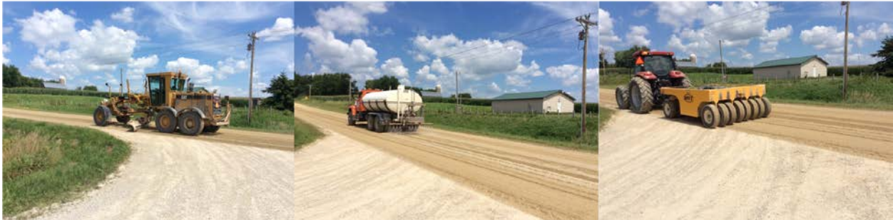
Figure 44. Chloride treatment at Goodhue County
