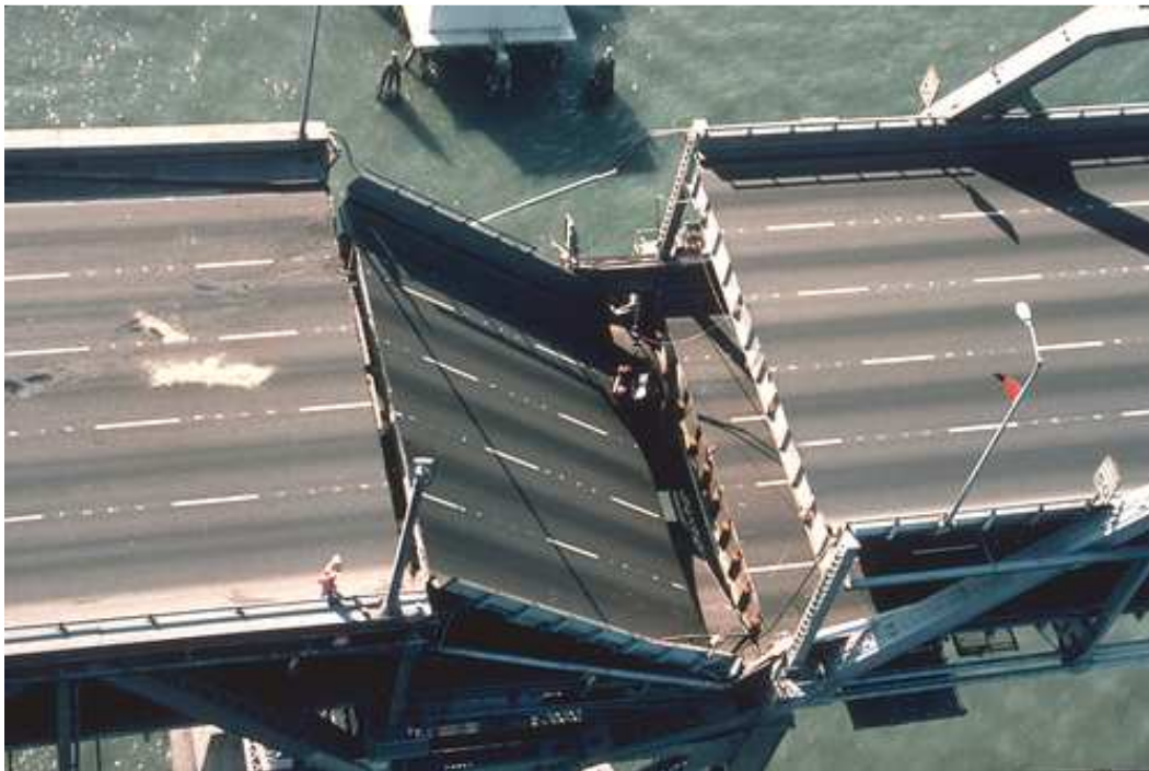
Figure 1.3. Bay Bridge collapse, 1989 (Eskenazi, 2009)
