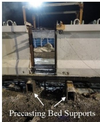
PPCB ends over the bed supports
