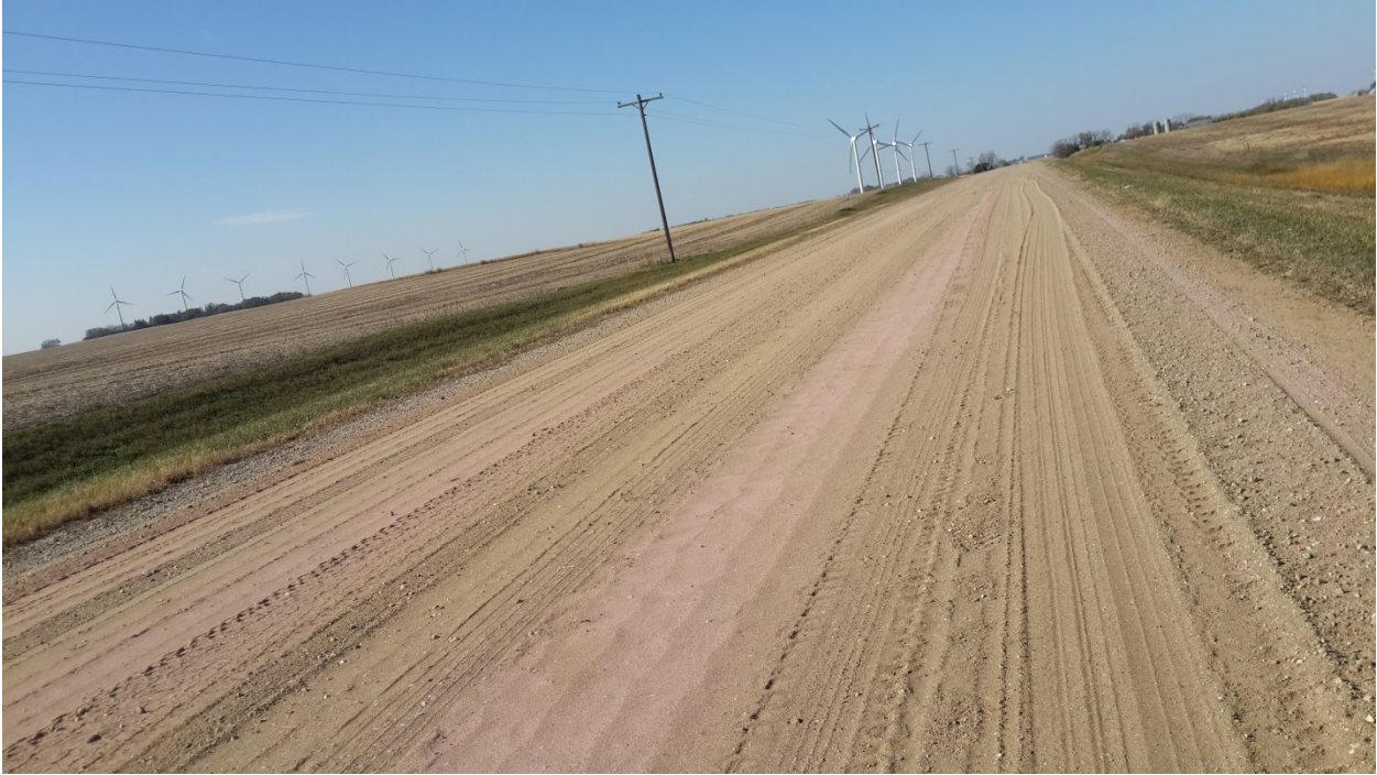
Figure 28 Jackson County Road 76 East Test Section (Photo by the Author)
