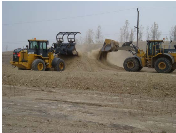
Figure 8 Stockpile Blending (Ted Eggebraaten and Ken Skoreth 2012)
