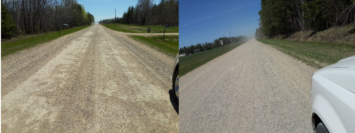
Figure 60 North Section (Left) and Middle Section (Right) (Photo by the Author)
