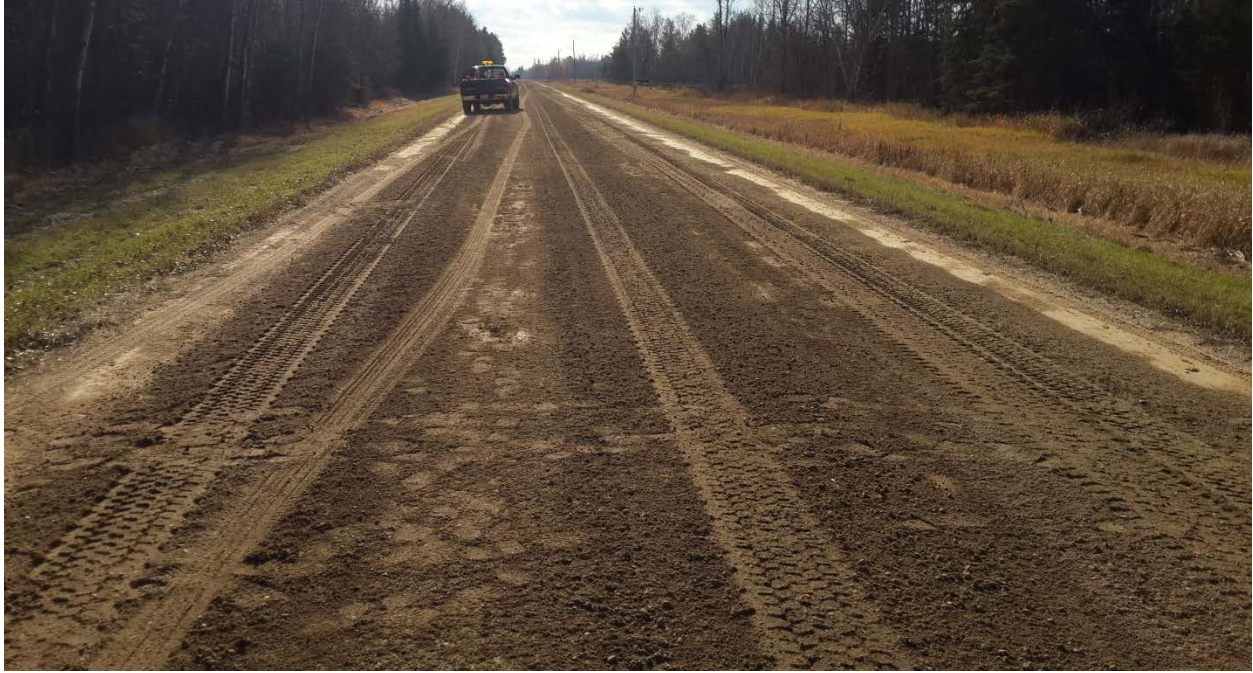
Figure 33 Beltrami County Road 23 North Test Section (Photo by the Author)
