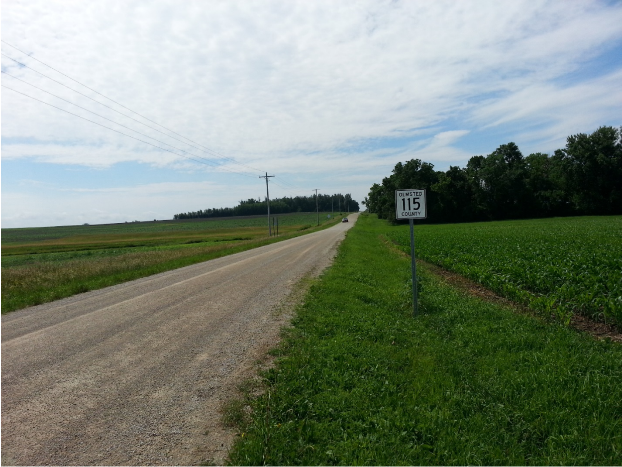
Figure 24 Olmsted County Road 115 Surface Conditions in July (Photo by the Author)
