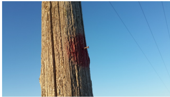
Figure 16 Red-Painted Benchmark on Power Pole (Photo by the Author)
