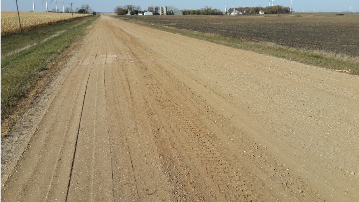
Figure 30 Jackson County Road 76 West Test Section (Photo by the Author)
