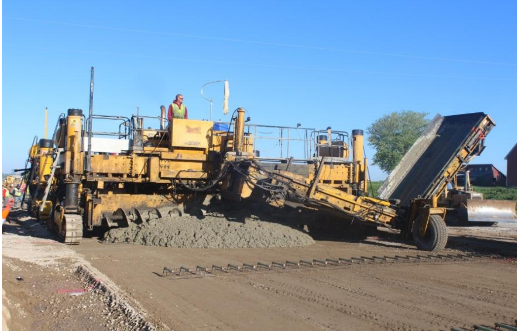
Figure 3-18. Concrete paving.
