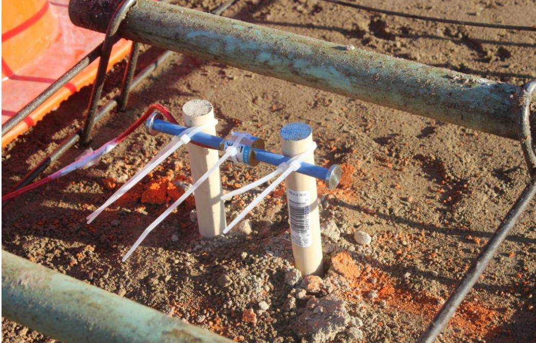
Figure 3-12. Installation of strain gage at joint.
