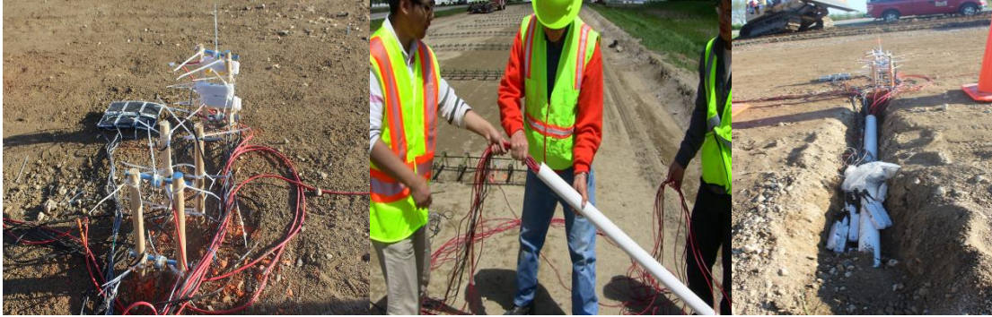
Figure 2: Sensor instrumentation on US-30 highway section
