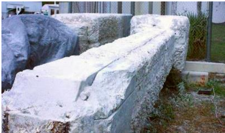
Figure 8. Actual vertical and horizontal saw cuts. (Bridge A Pile #2)
