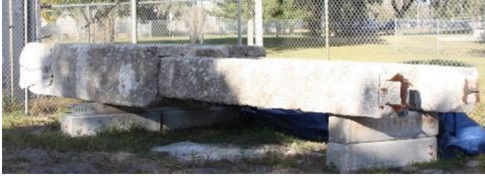
Figure 1. Bridge A piles resting side-by-side on horizontal concrete columns. Note jackets on upper area (left) of piles and H-beams visible at each pile bottom end (right).
