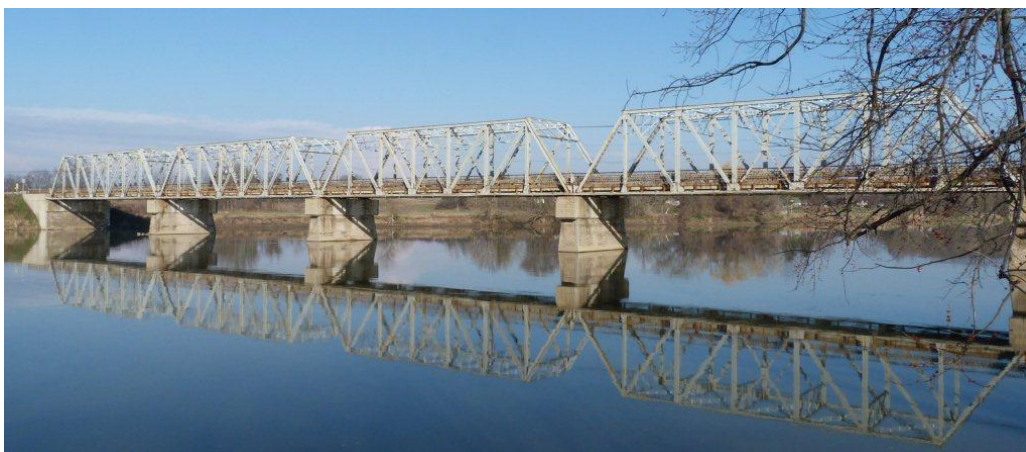
Figure C.10.1 Highway 3 Grand River Bridge Current Condition
