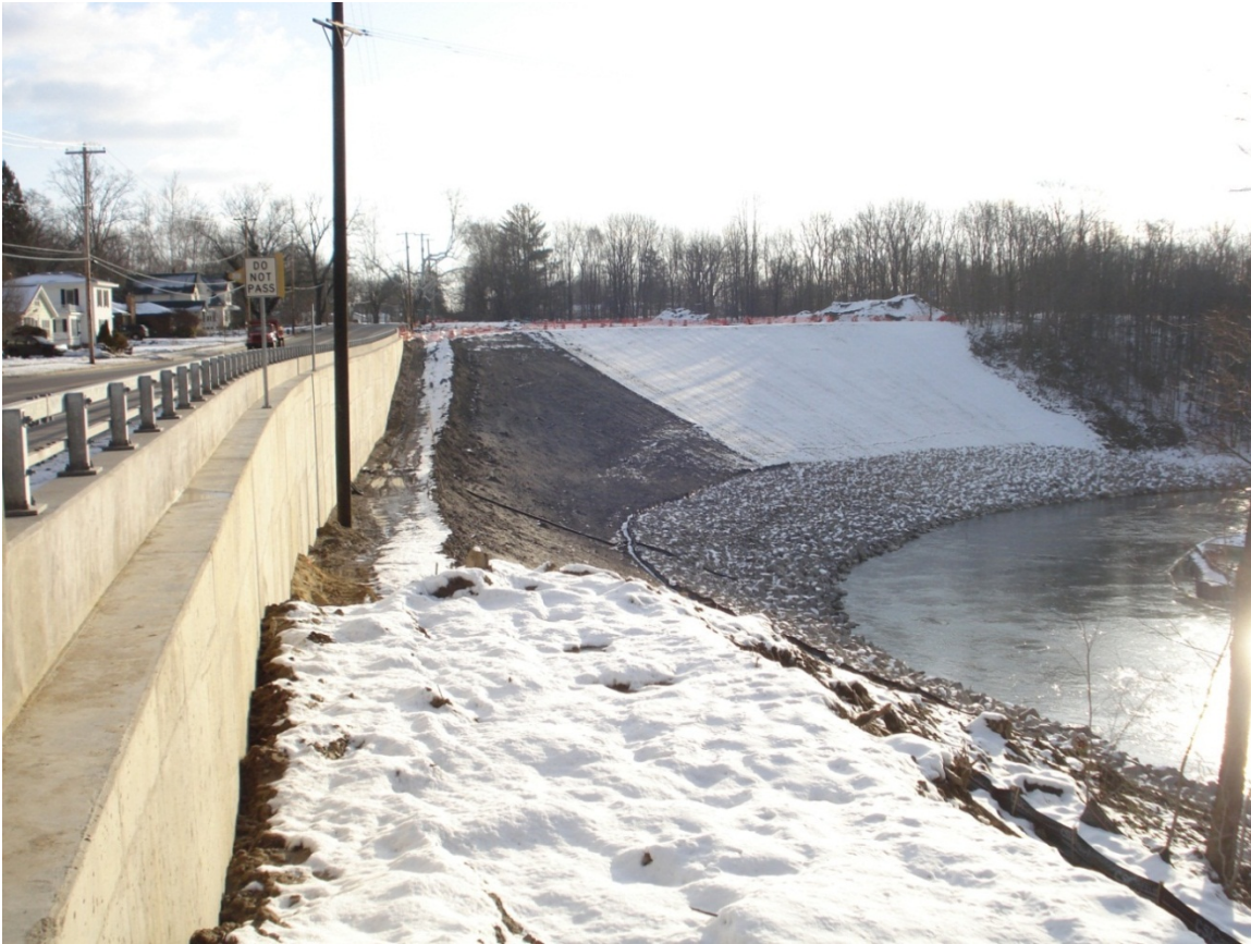
Figure C.4.1 M-222 Slope Stabilization post construction. Photo courtesy of MDOT.
